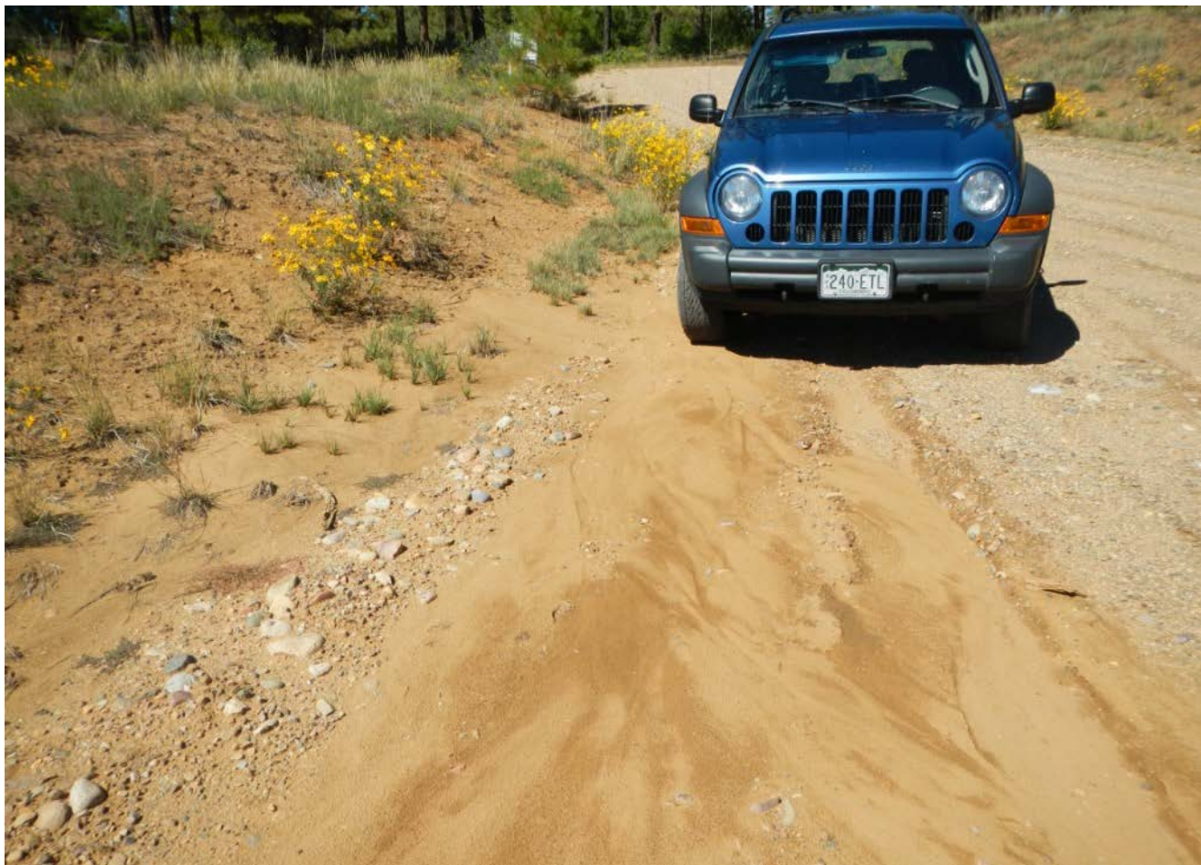
Photo 5. View of sediment run-on from the western edge of the access road near the entrance to the well pad.
