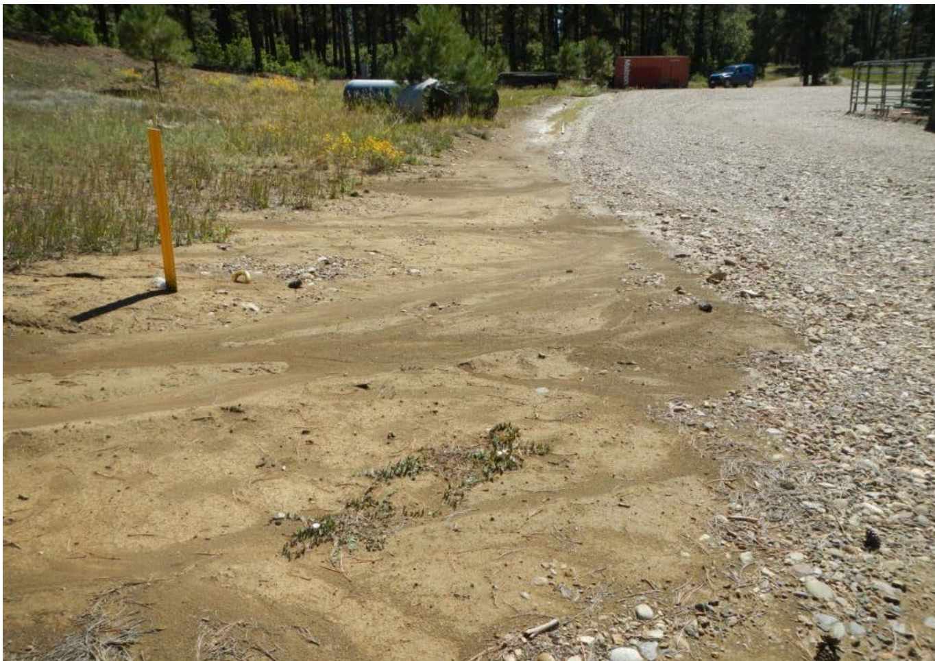
Photo 4. View of sediment deposition on the well pad at the base of the cut slope shown in Photo 3. Sediment appears to be contained but erosion needs to be monitored.
