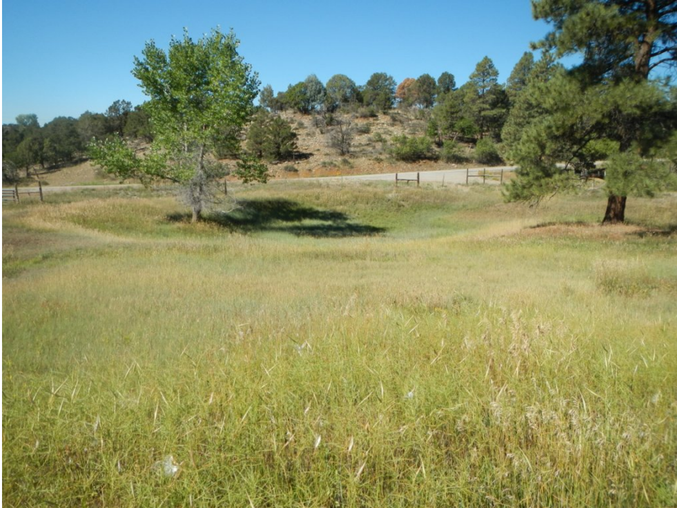
Photo 4. View of vegetated swale and silt trap within western portion of interim reclamation area.
