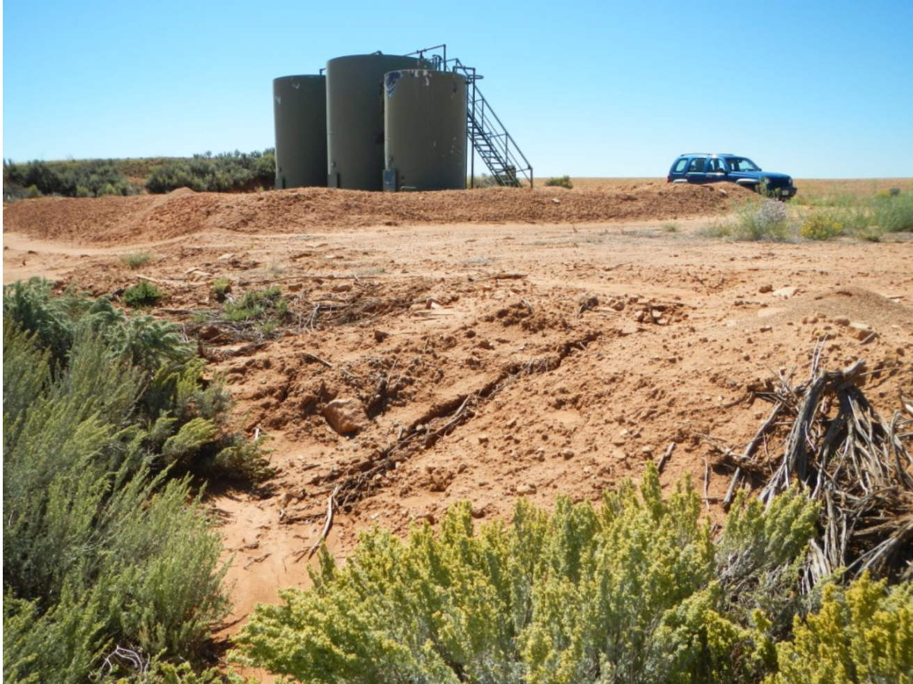
Photo 3. View of rill erosion on eastern edge of well pad.
