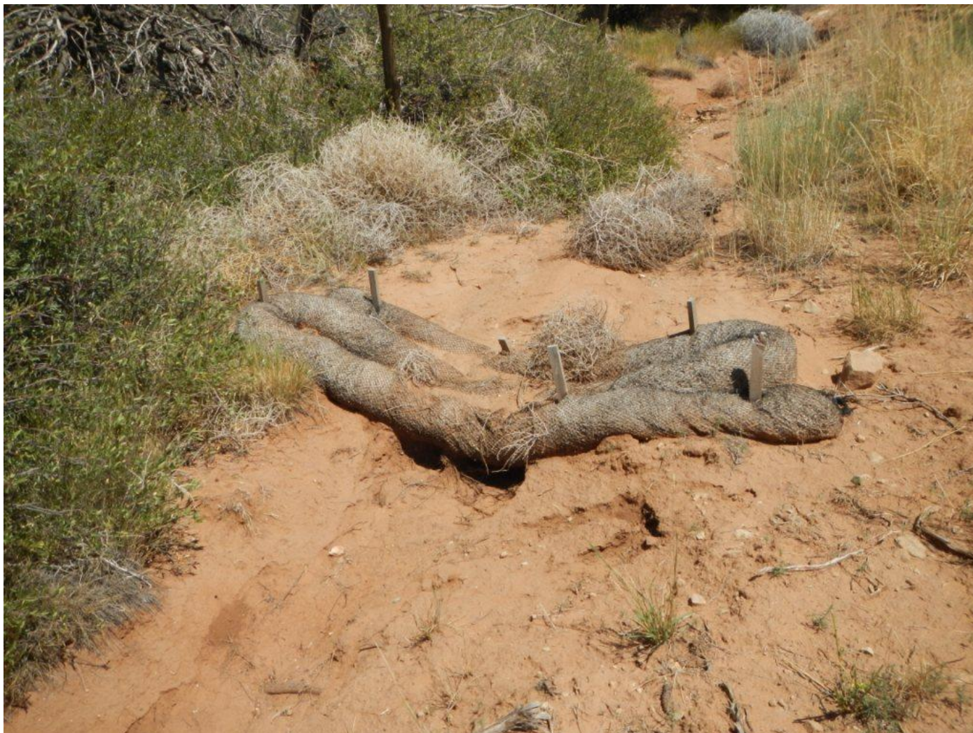
Photo 4. View of failed straw wattle on northern side of access road, downstream of well pad and rock check dams.
