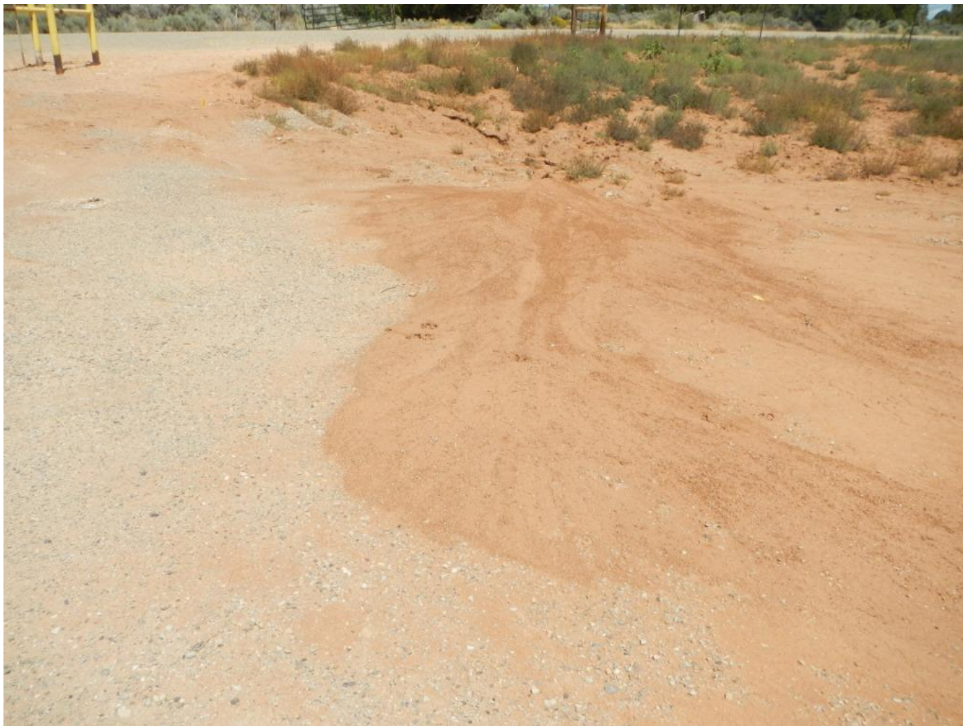
Photo 5. View of sediment discharge onto the well pad adjacent to the access road at the entrance to the well pad.
