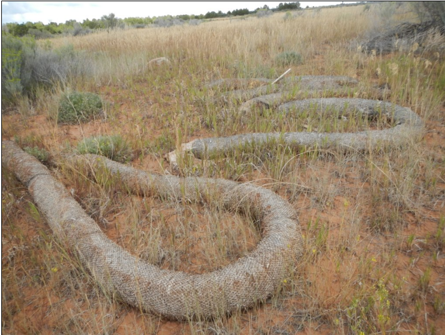
Photo 5. View of unused straw wattles that need to be properly installed or removed from project area.
