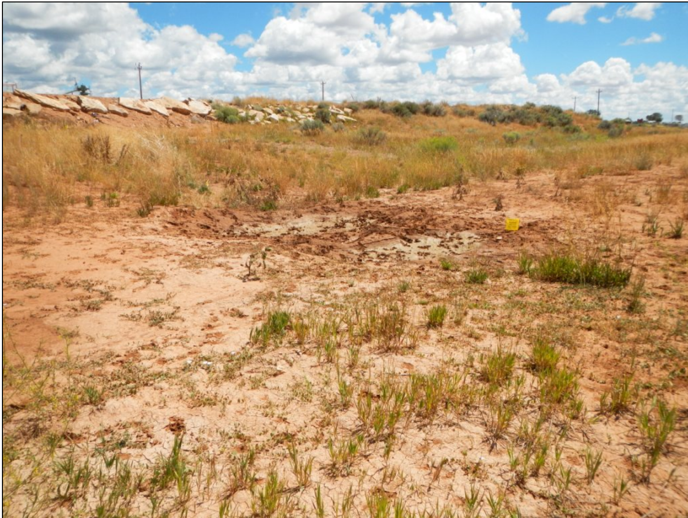
Photo 3. View of silt trap in western portion of interim reclamation area that is filling with sediment.
