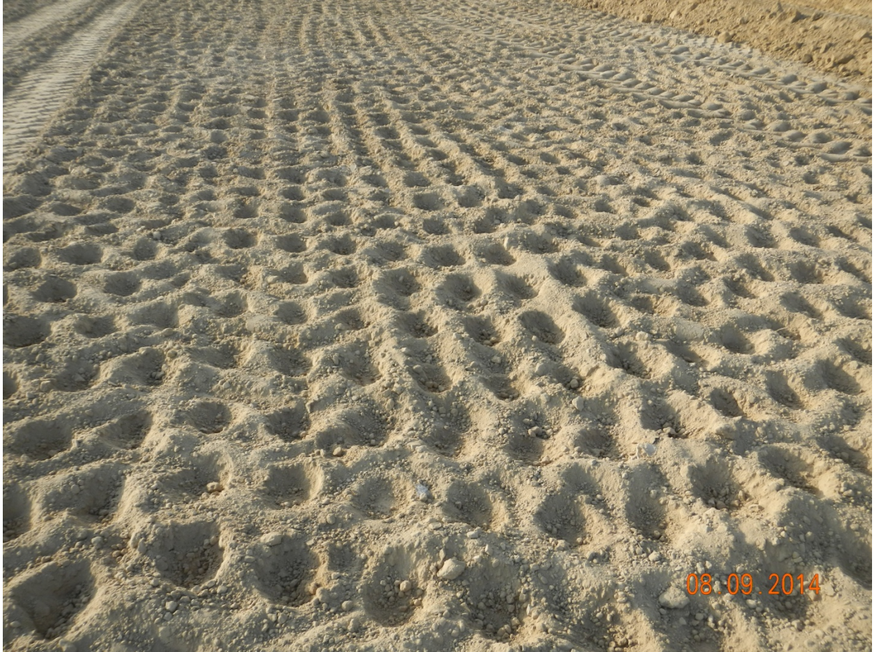
16. Sheep-foot surface roughening on fill areas of location.
