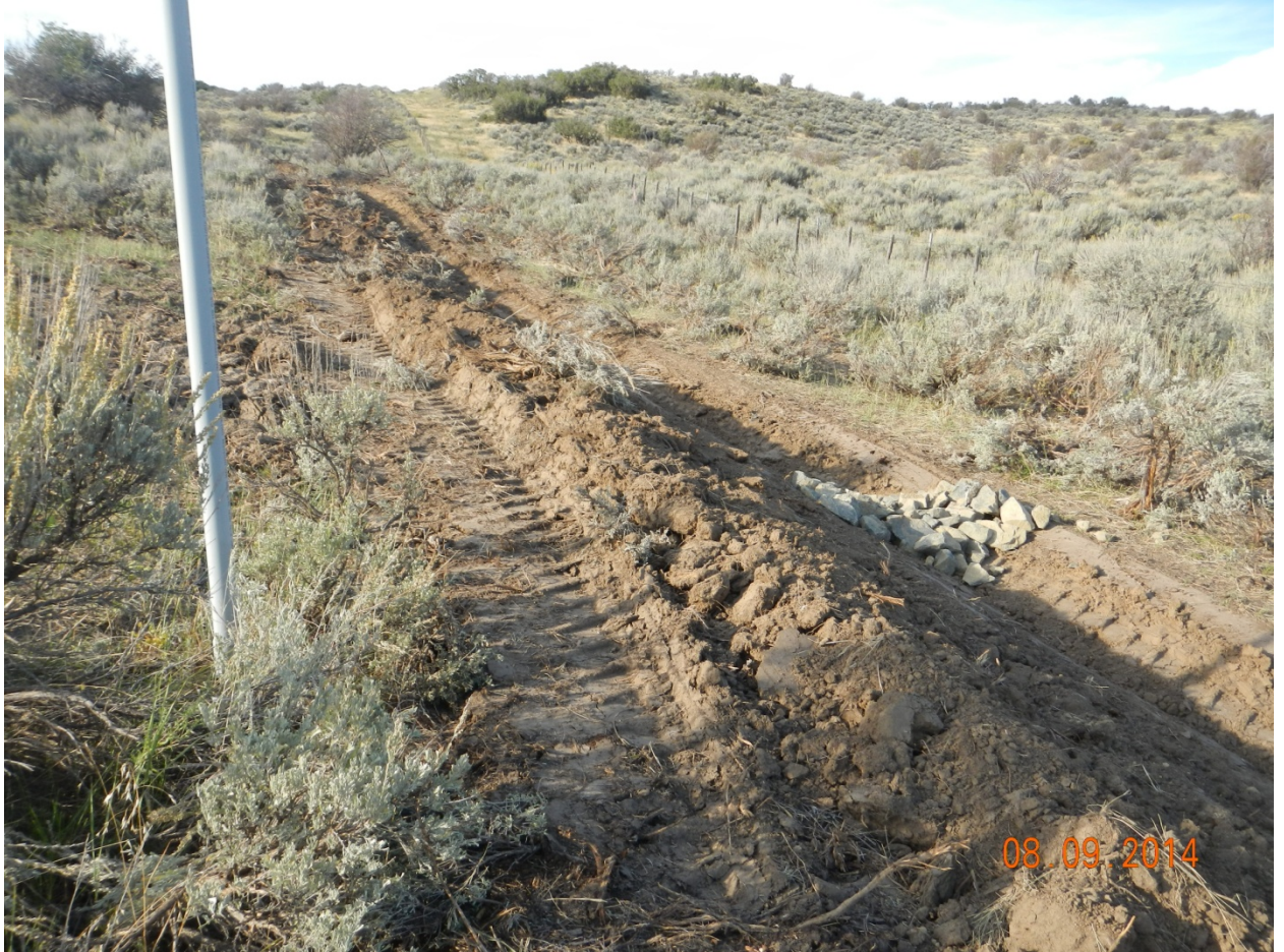
10. Diversion above North cut tracked with stormwater check-dams.
