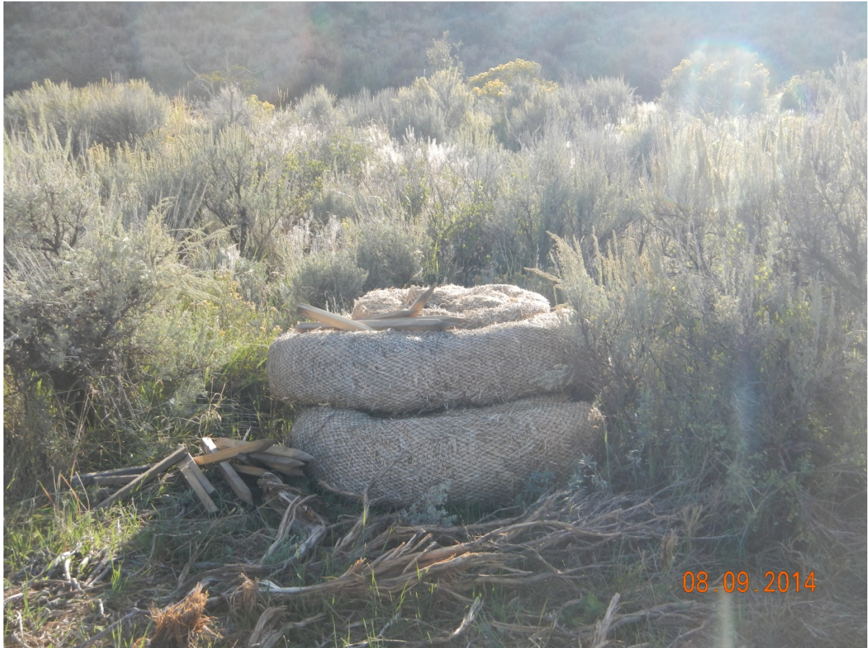
17. Waddles on West perimeter yet to be installed.
