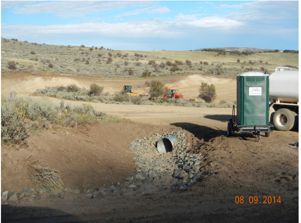
4. Entrance stormwater bmps performing (1).
