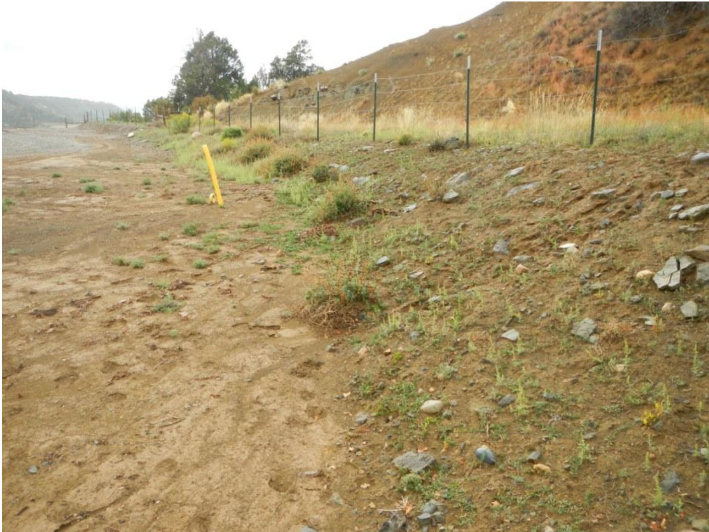
Photo 3. View of western edge of the well pad. It appears that sediment is eroding from adjacent slopes.
