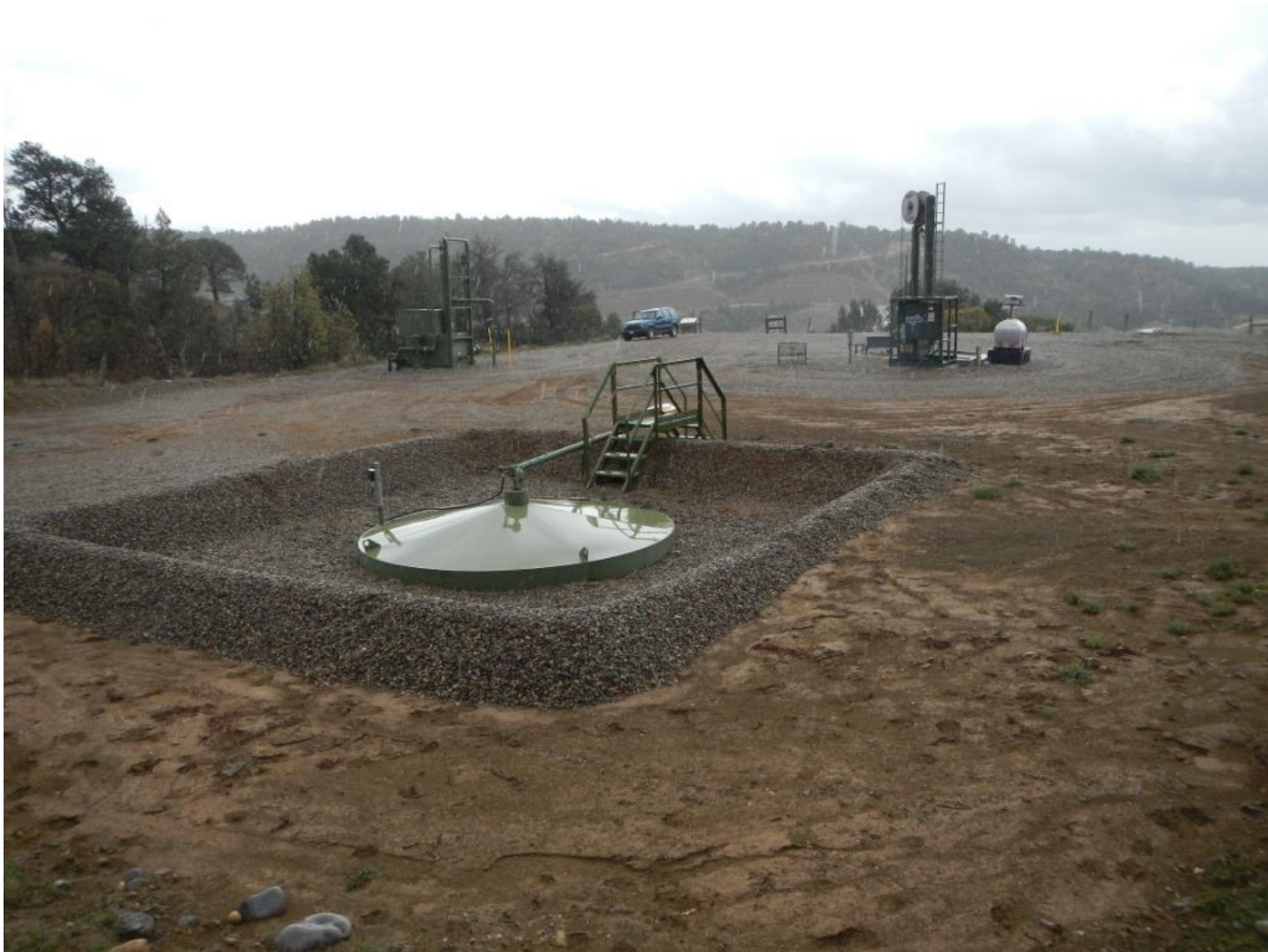
Photo 2. View from northwestern corner of well pad facing center. It appears that sediment in the foreground has eroded from adjacent (north and west) slopes.
