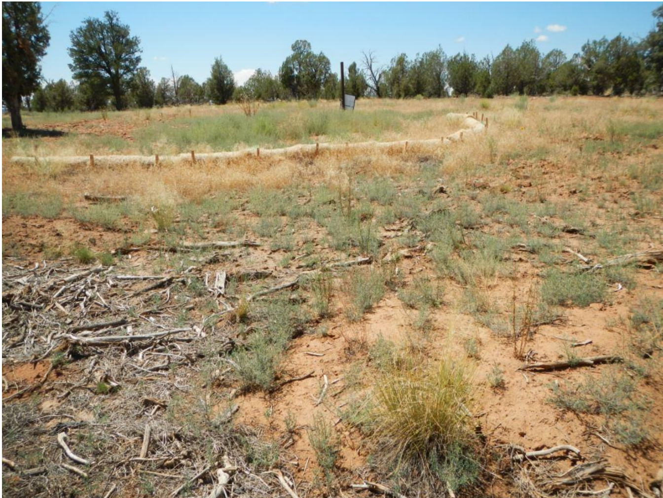
Photo 1. View from northeastern corner of well pad toward center. Straw wattle appears to be functioning properly.
