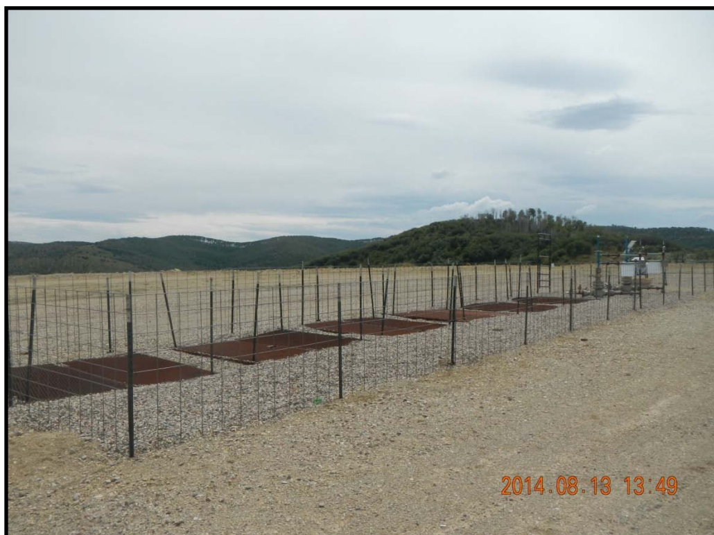
Two active wells and six conductors. Fenced. No staining observed.
