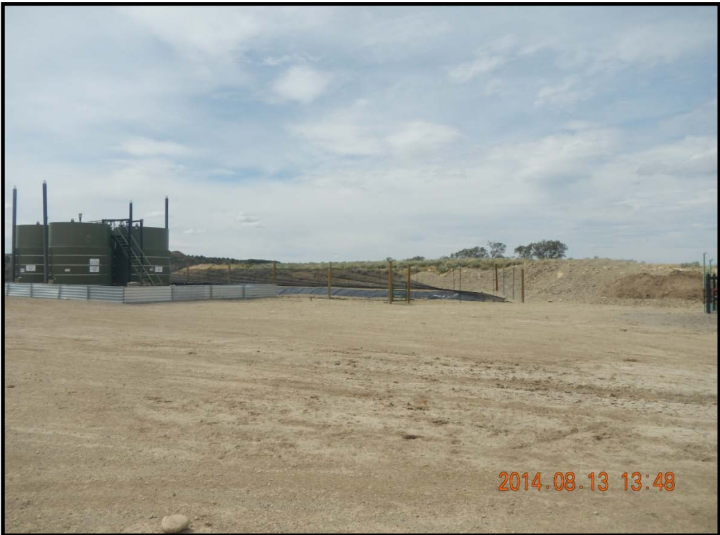
Bermed Tank Battery, and stockpile.
