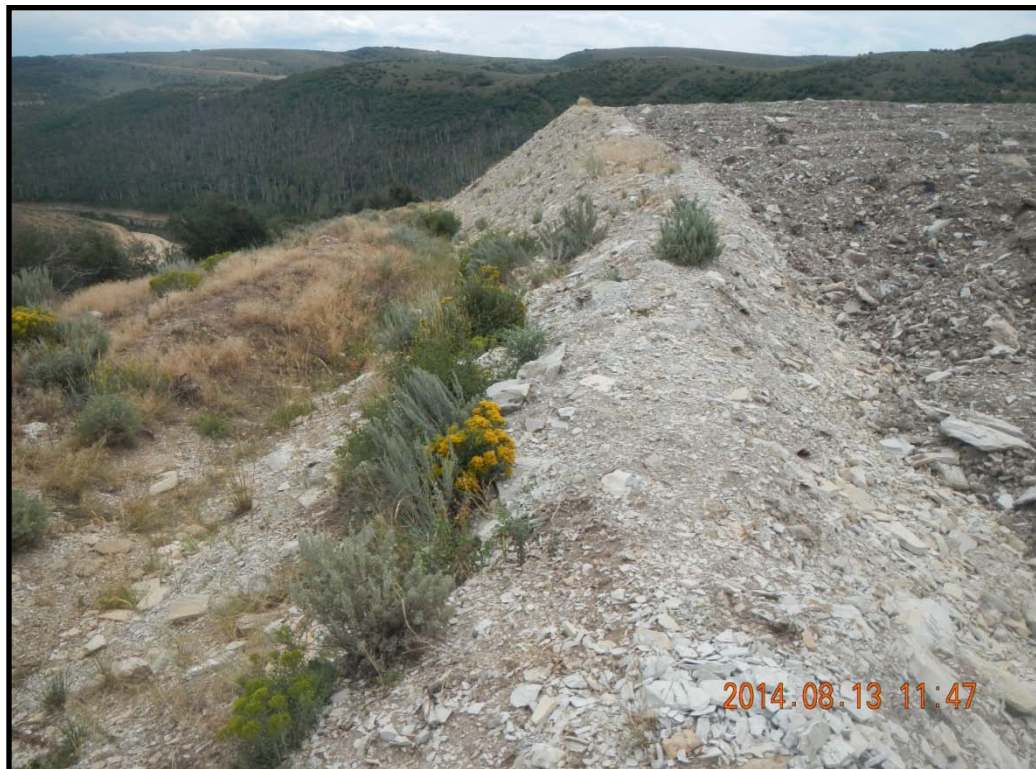
Berm around the landfarm operation.
