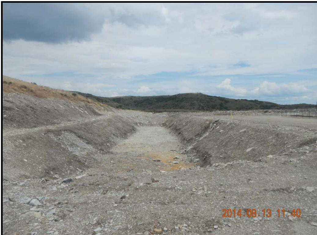
Pit Facility ID # 423848. Pit empty. Liner removed. Bottom of pit has been excavated and material extended in site for landfarming. No signs of staining in the pit.
