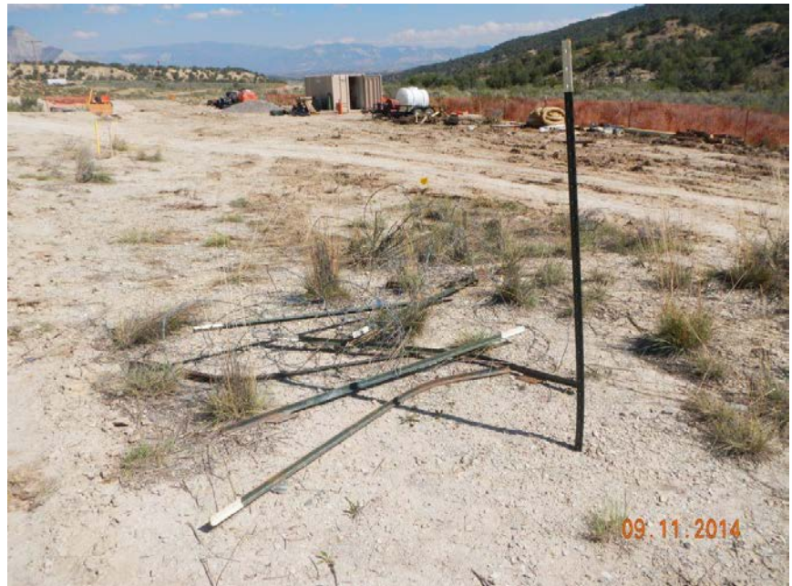
Fencing material to be removed
