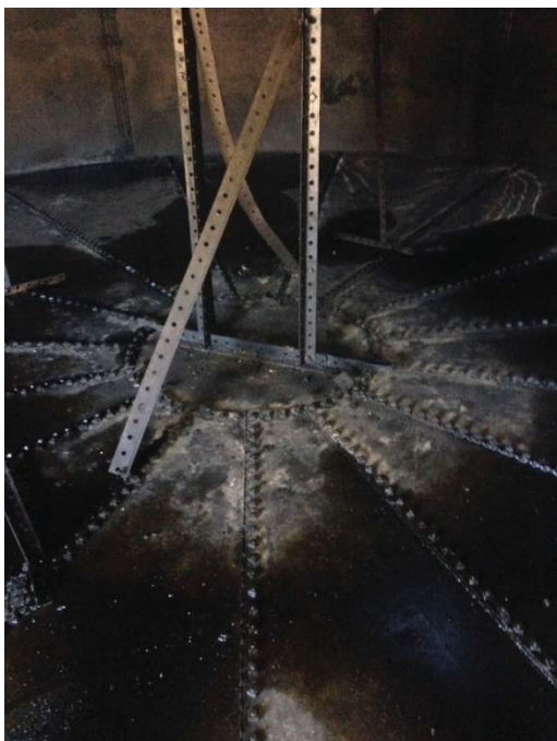
Figure 5 – Brace in Tank 4
