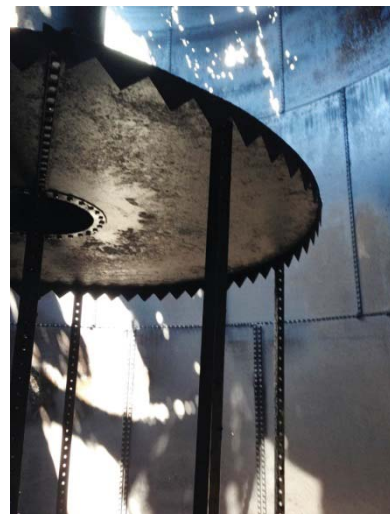
Figure 6 – Down comer in Tank 4
