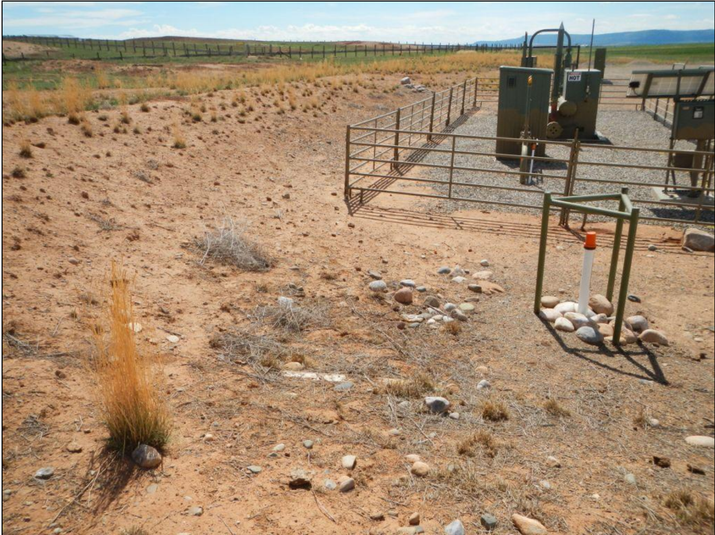
Photo 3. View of sediment that has discharged off of the interim reclamation area slopes onto the working area in the northeastern corner of the well pad.
