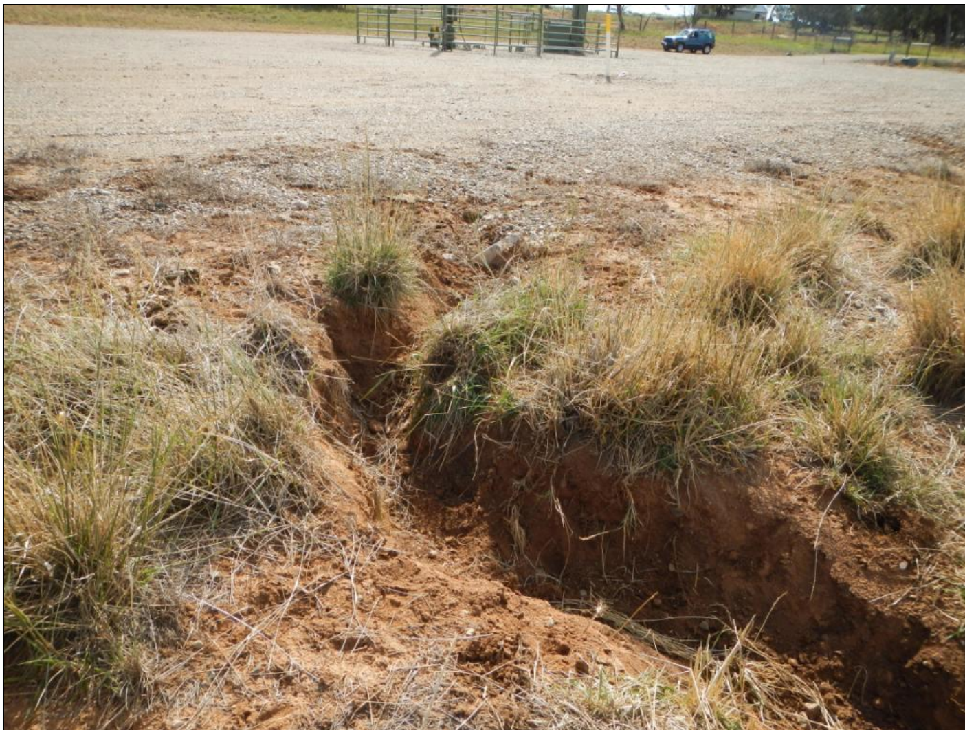
Photo 3. View of erosive feature on the western edge of the well pad.
