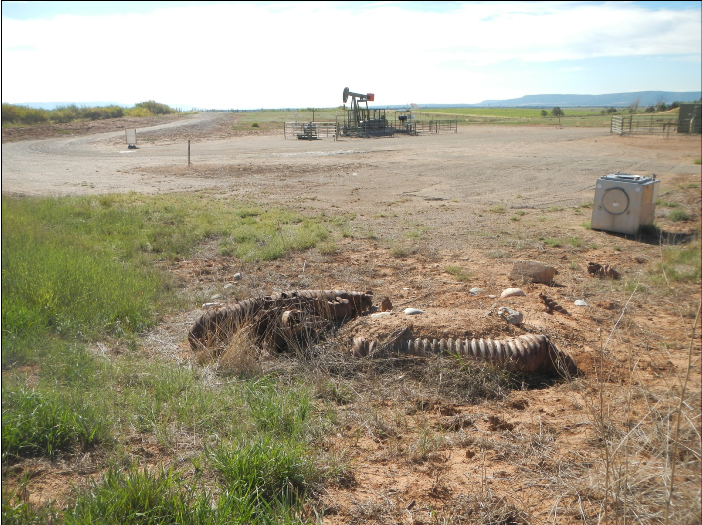
Photo 1. View of unused Tol-pac, damaged culvert, and debris in northwestern corner of well pad.
