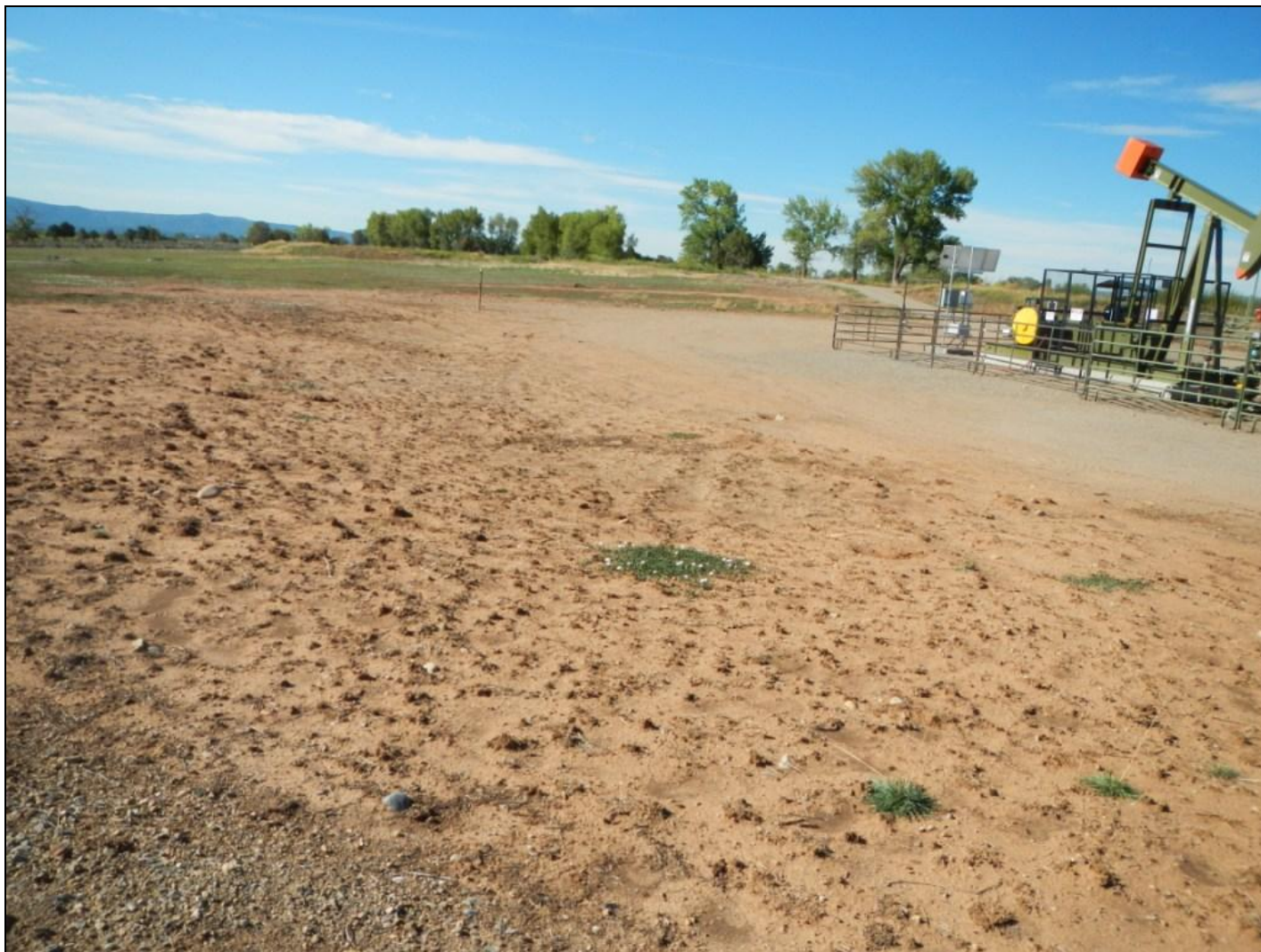
Photo 3. View of interim reclamation area from approximate northeastern corner of well pad facing southward. Run-on from unvegetated interim reclamation area onto well pad can be seen.
