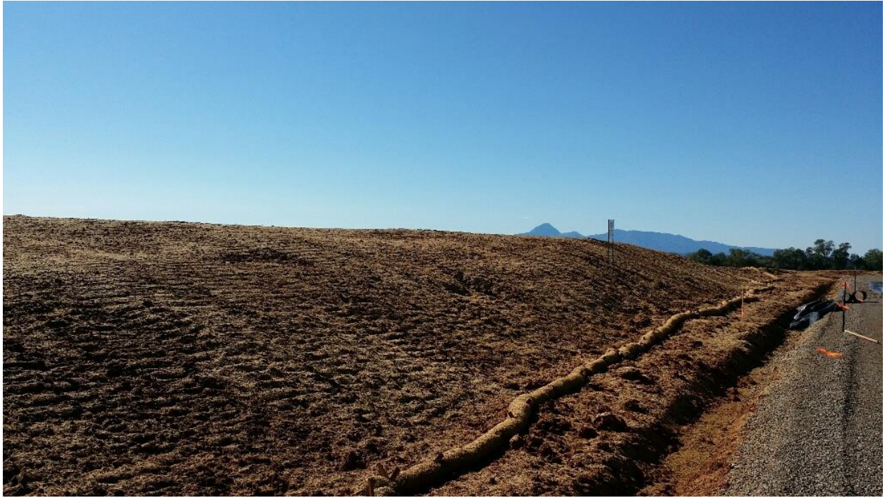
Topsoil stockpile stabilized
