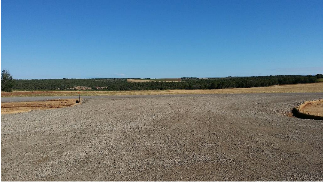
CB-3 access road stabilized to control any tracking of sediments.
