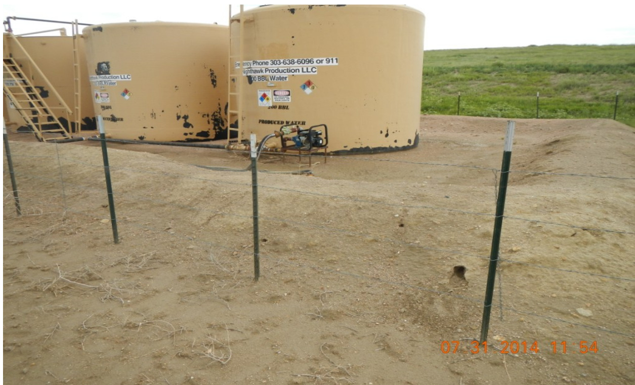
Photo #8 Rills off of slope on South side of location.
