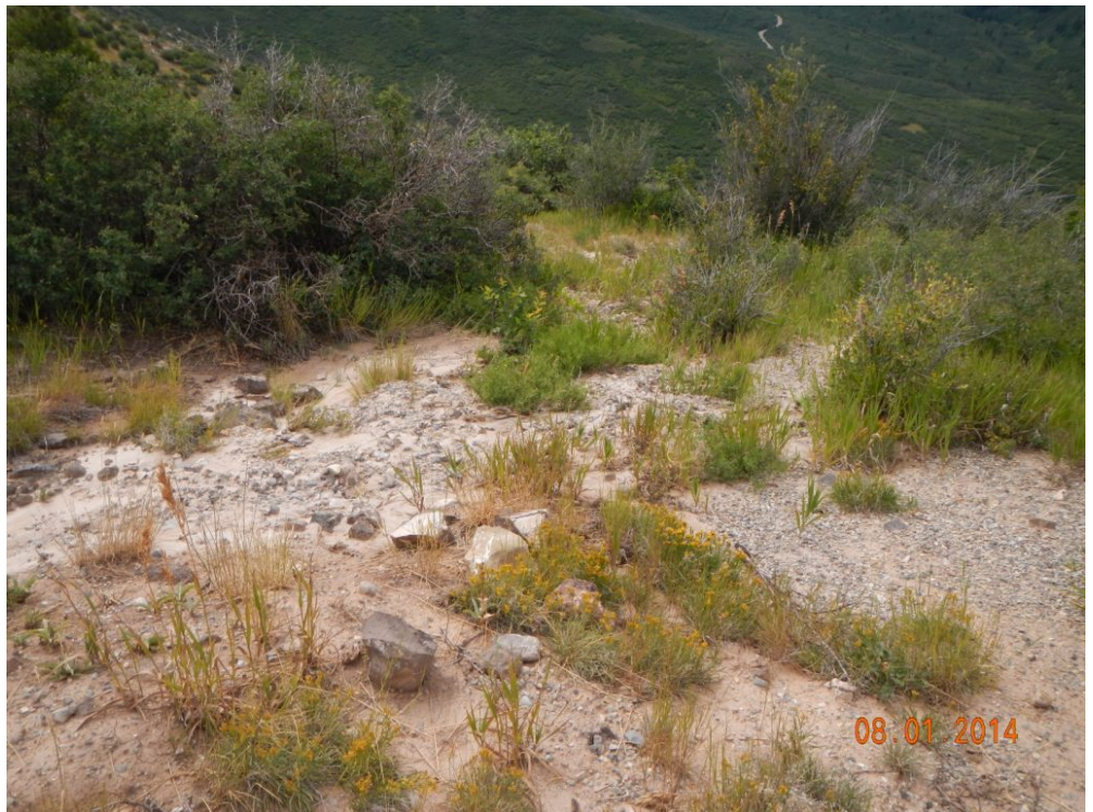
Sediment in vegetation from erosion on access road.
