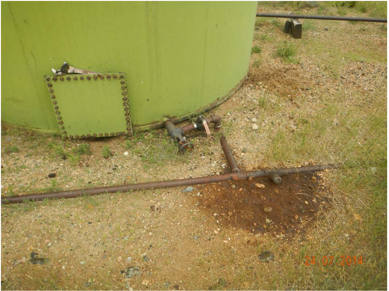
7.) Staining beneath oil filter remains
