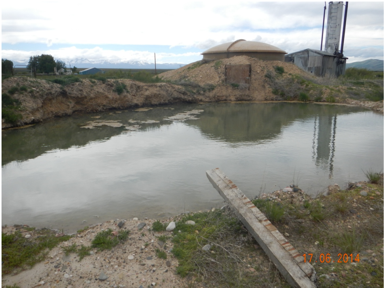
7.) Pit at less than 2 feet of freeboard.
