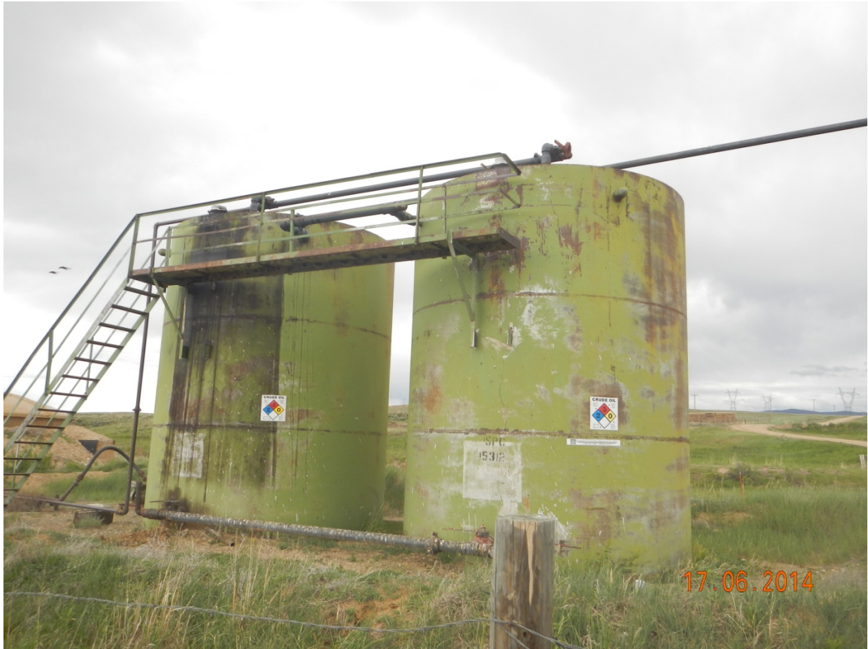
4.) Staining on tanks.
