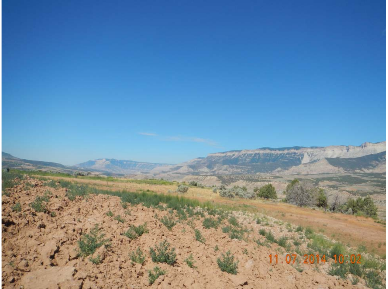
Surface roughening appropriate stormwater BMP. Vegetation sparse.
