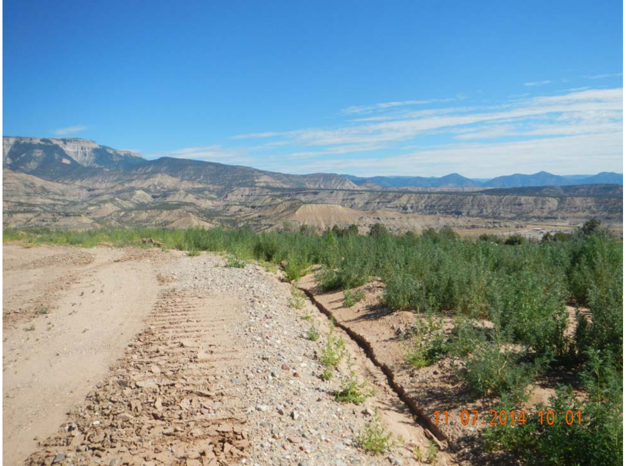
Erosion and rilling on Northern pad perimeter.
