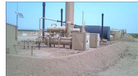
SEPARATORS, METERS, AND EMISSION CONTROL DEVICE CONTAINMENT BERM (TYP)
