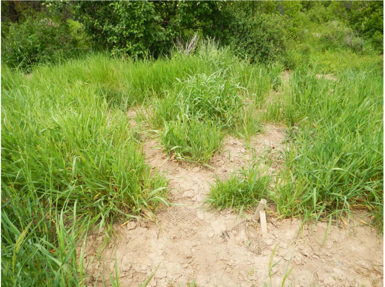
Perimeter wattles failing (1)
