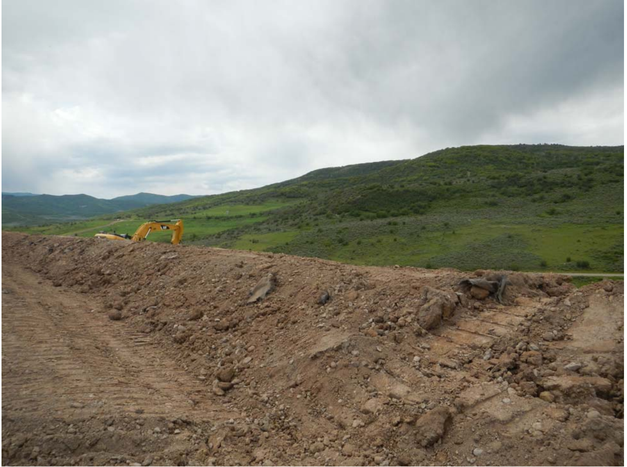
Debris being incorporated into perimeter berms
