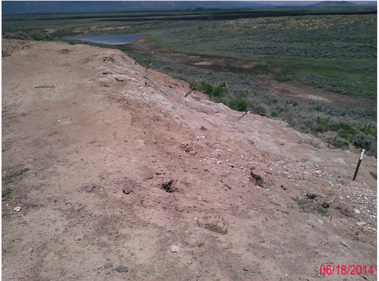
Sediment run-off, by pit and fencing down (2).
