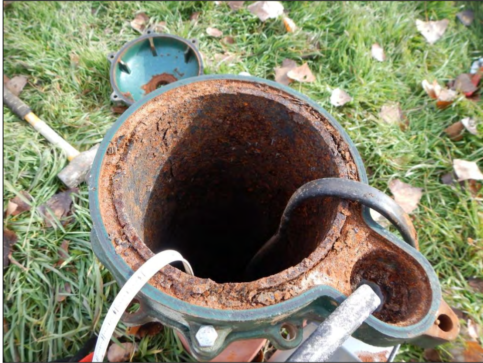
Photo 7. Water Well Permit No. 276703 Sampling Location (Palmer 276703), View Inside Rusted Well
