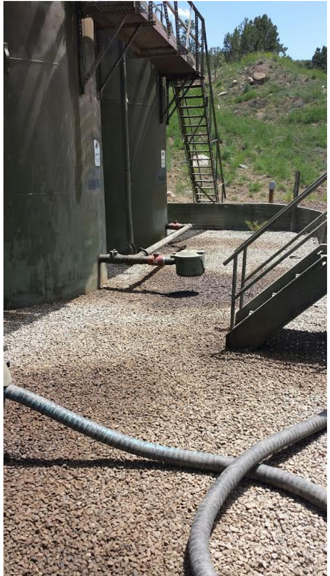
Staining on tanks and on ground.
