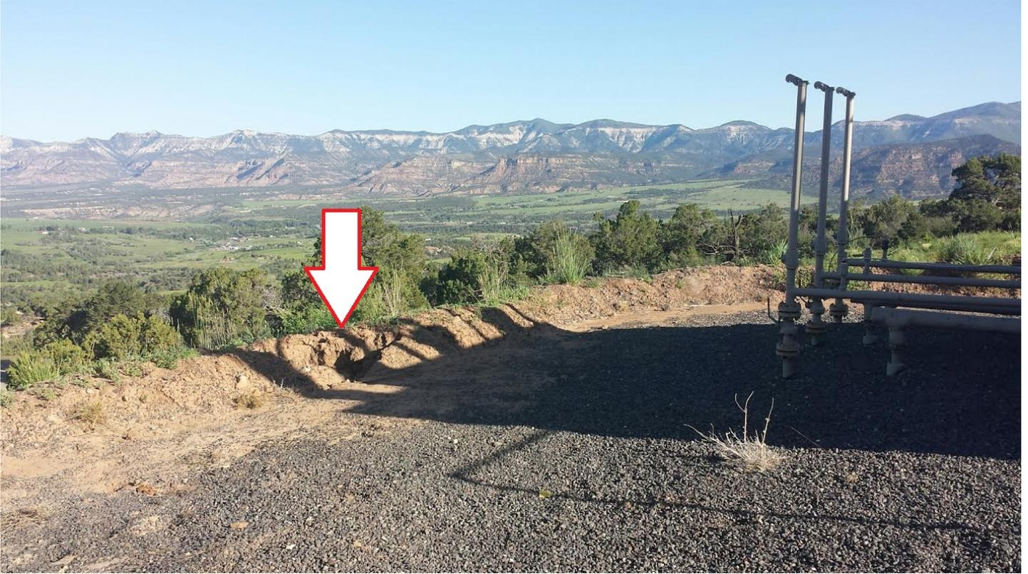
Breach in berm behind separators.
