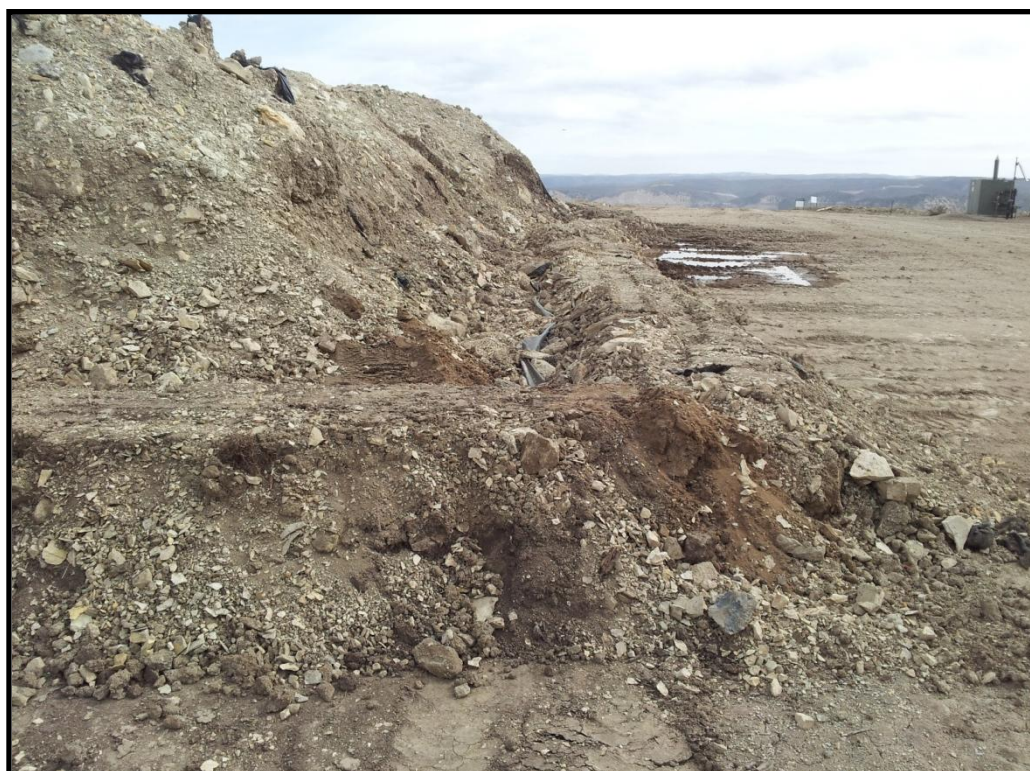
Fluids seeping through the berm.
