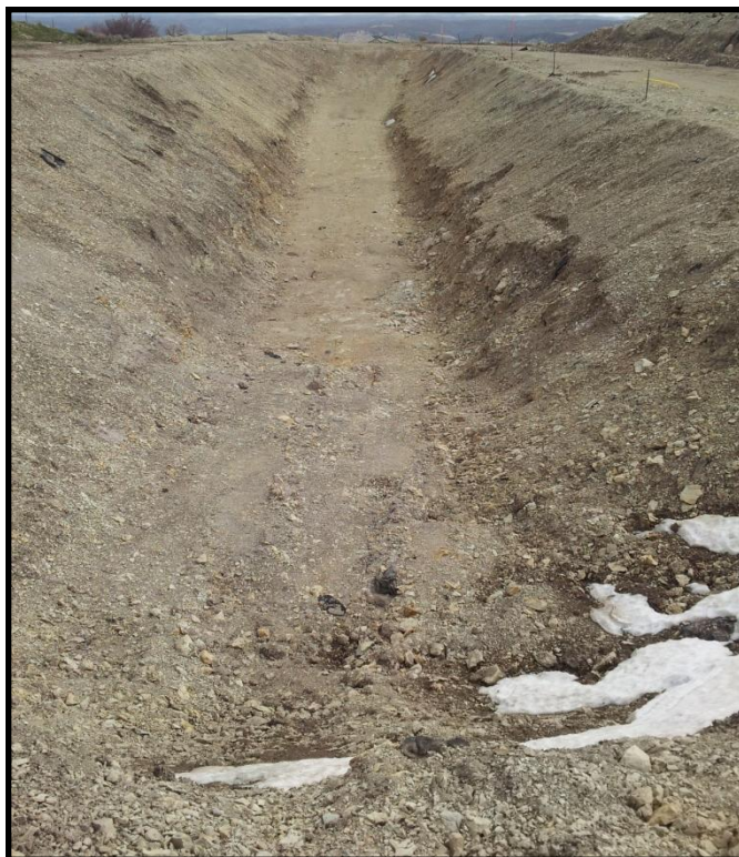
Pit excavated. Some trash on the walls (pieces of liner).
