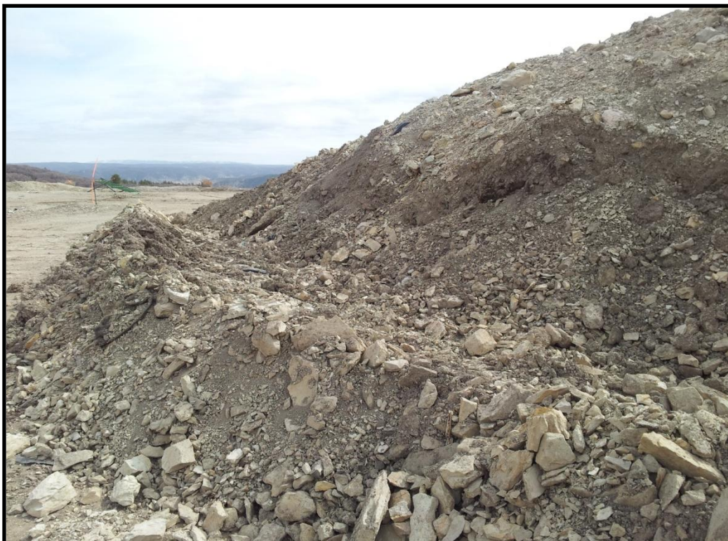
Berm apparently made of the same material excavated from the pit
