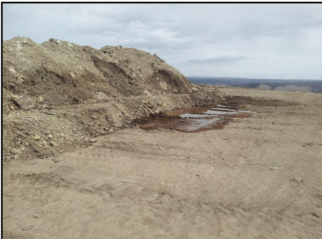
Fluids seeping through the berm.
