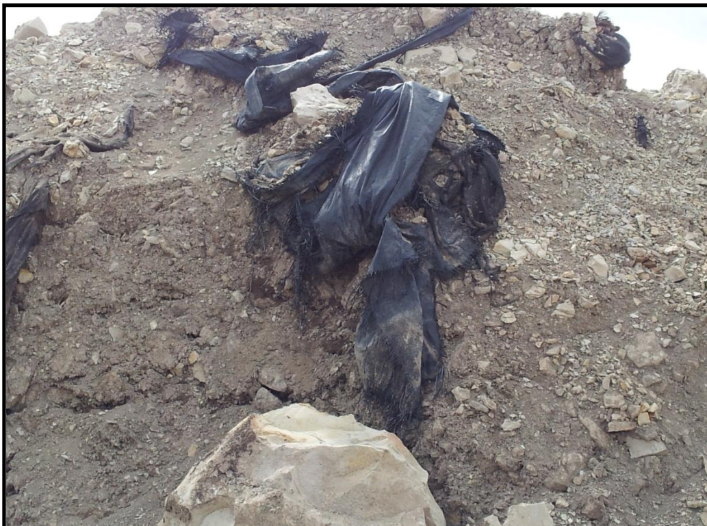
Pieces of liner mixed with the stockpile material.
