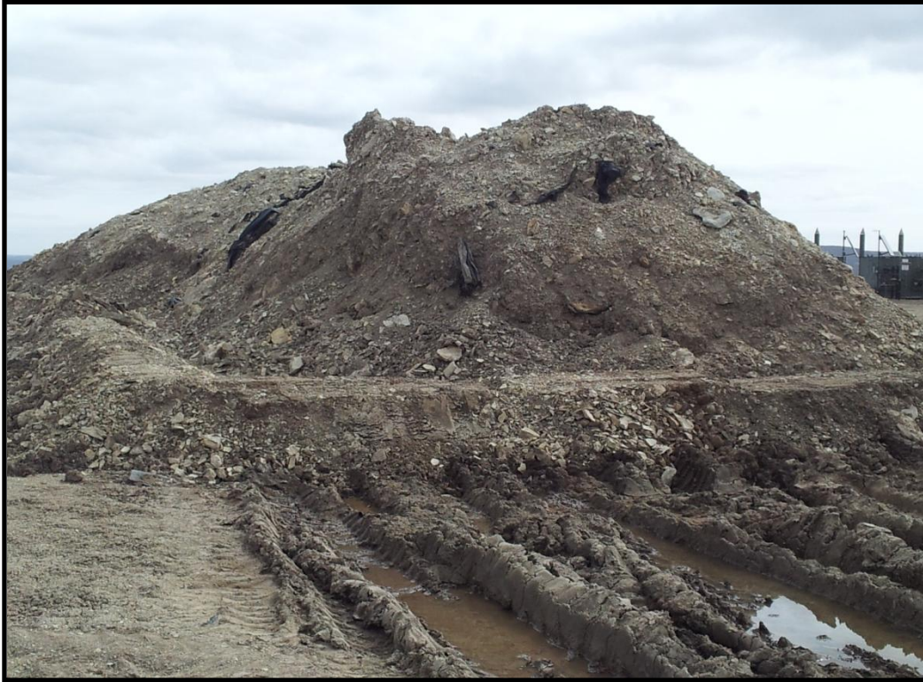
Stockpile with material from the pit. Fluid from the stockpile seeping through the berm. Pieces of liner mixed with the material.
