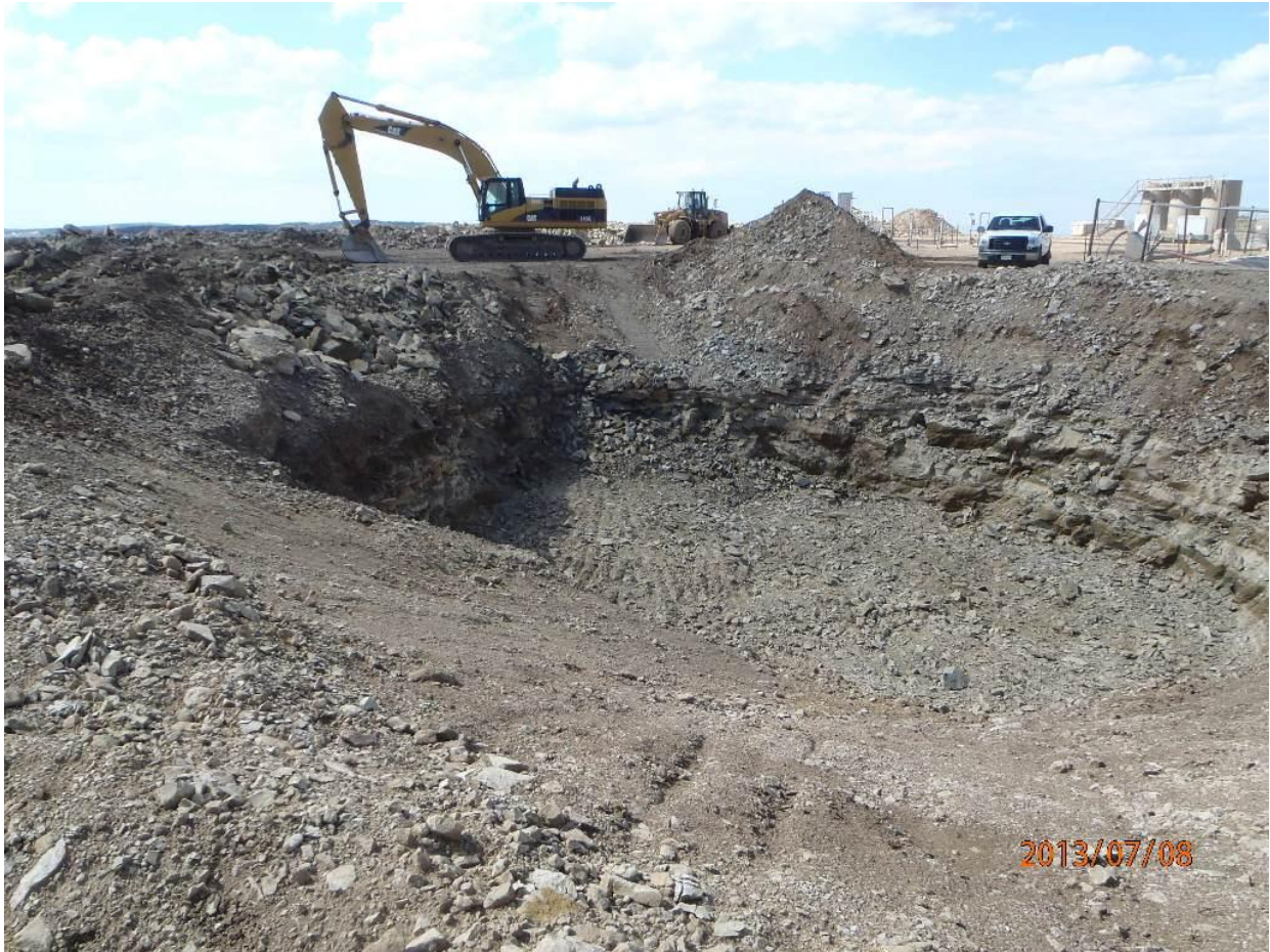
Visual representation of the soils on pit bottom and pit walls post excavation
