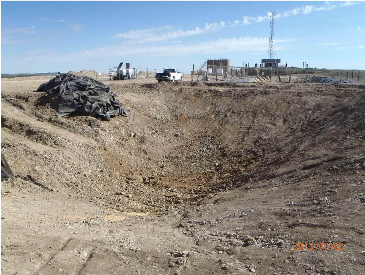
Visual representation of the impacted soils on pit bottom and pit walls prior to excavation
