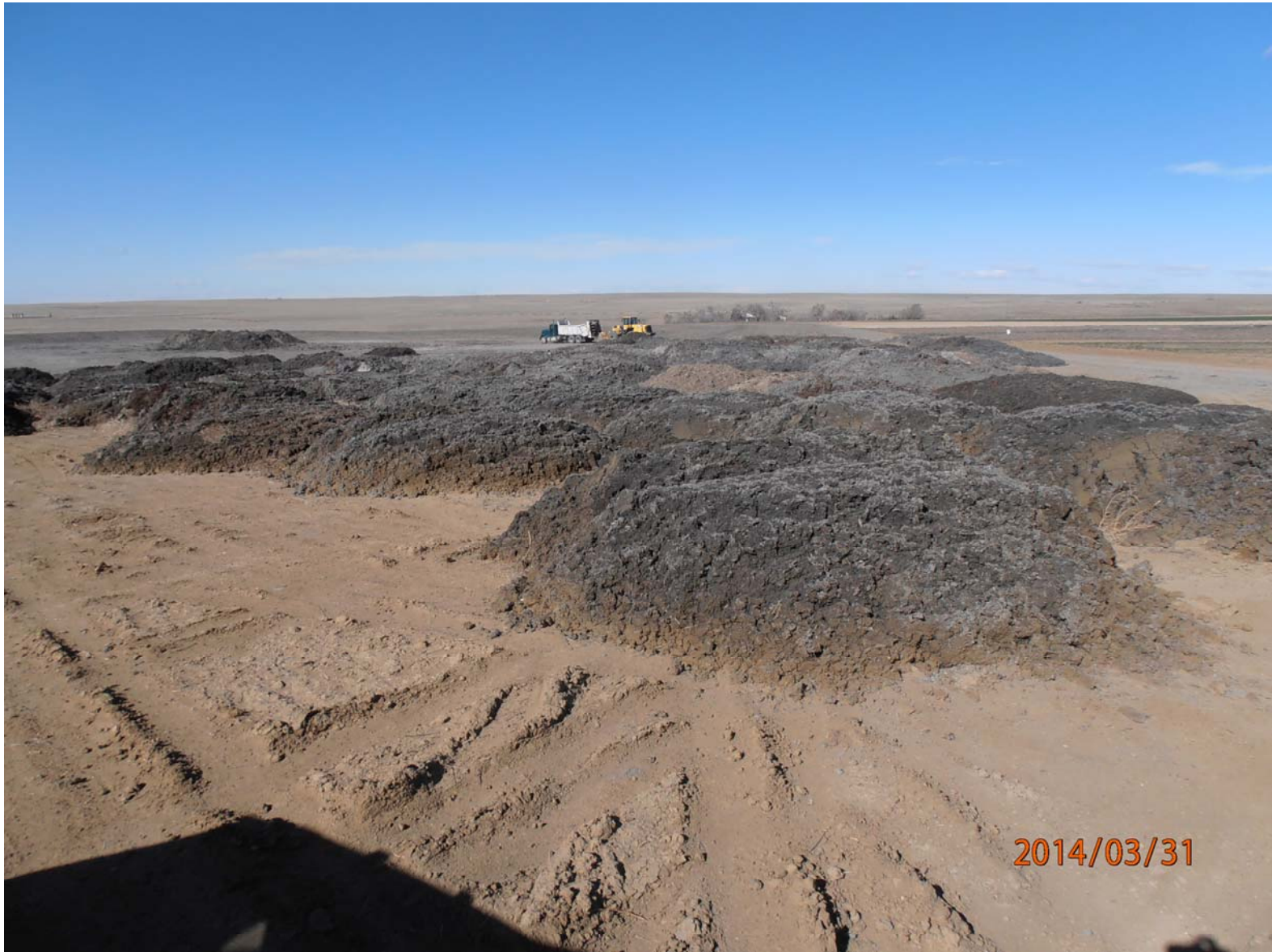
Photo at Stockpile area 2 looking west toward stockpile 1
