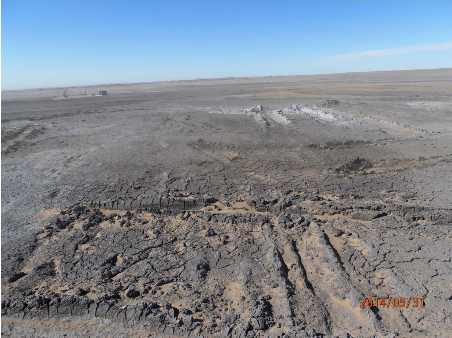
Photo at stockpile area 3, looking southwest; evidence of ponded and evaporated fluid
