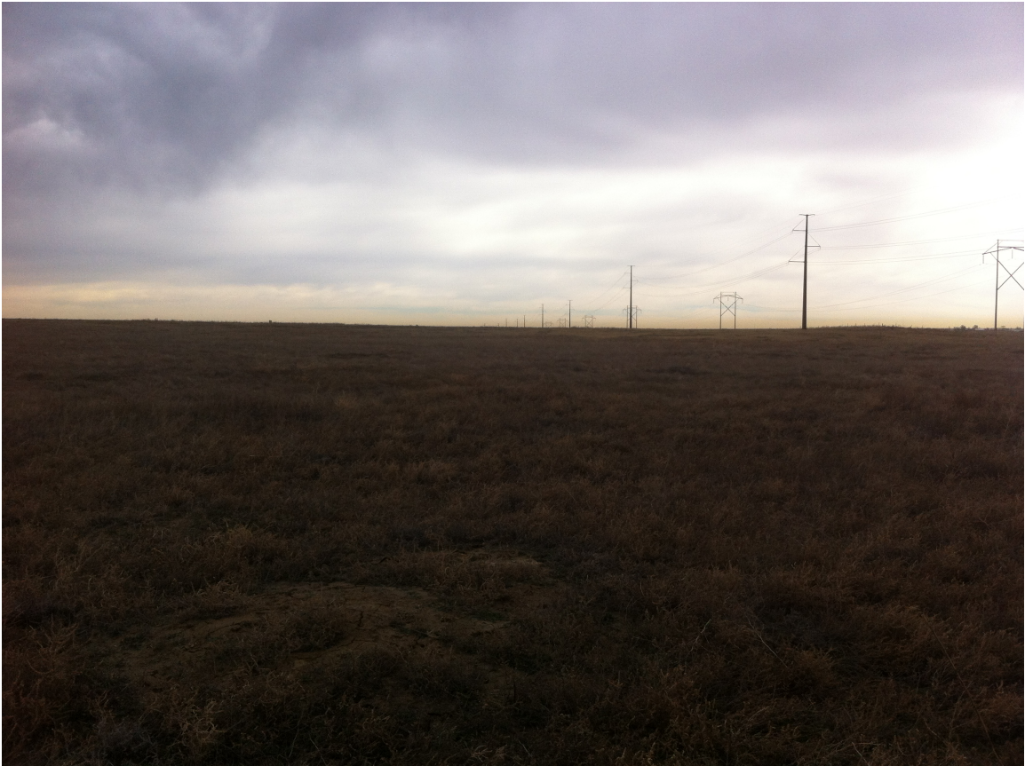
DOLPH TANK BATTERY 1N-1HZ
