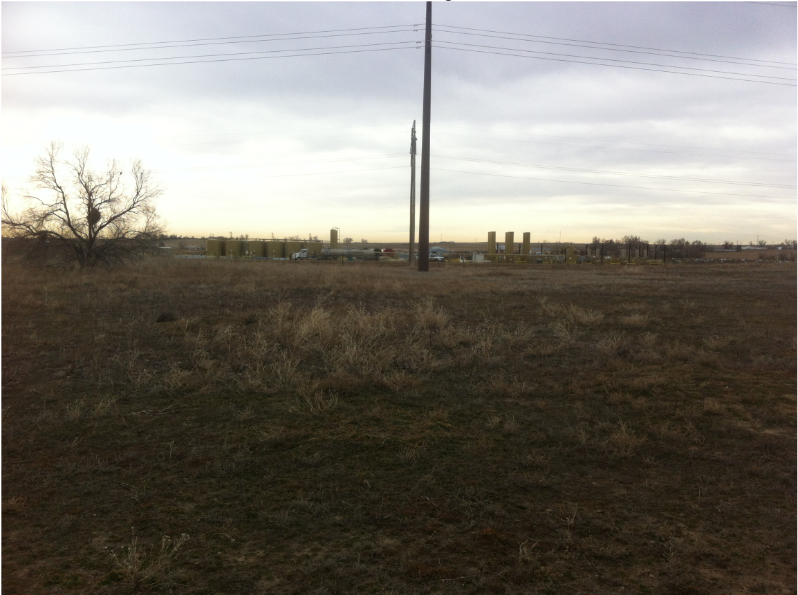
DOLPH TANK BATTERY 1N-1HZ
