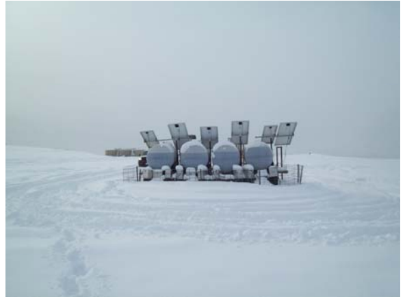
PAD LOCATION LOOKING SOUTH
