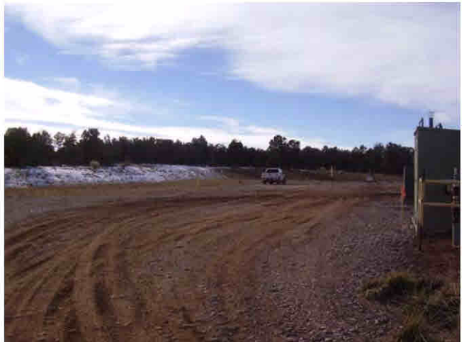
Access at Road
