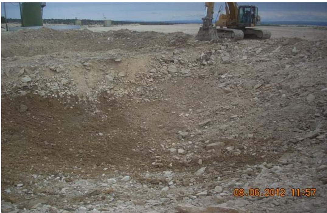
Photo 4 – View of the western end of the pit after removal of the contaminated soil. Photo is taken from the northwest corner looking southeast. Photo taken on 8/6/2012.
