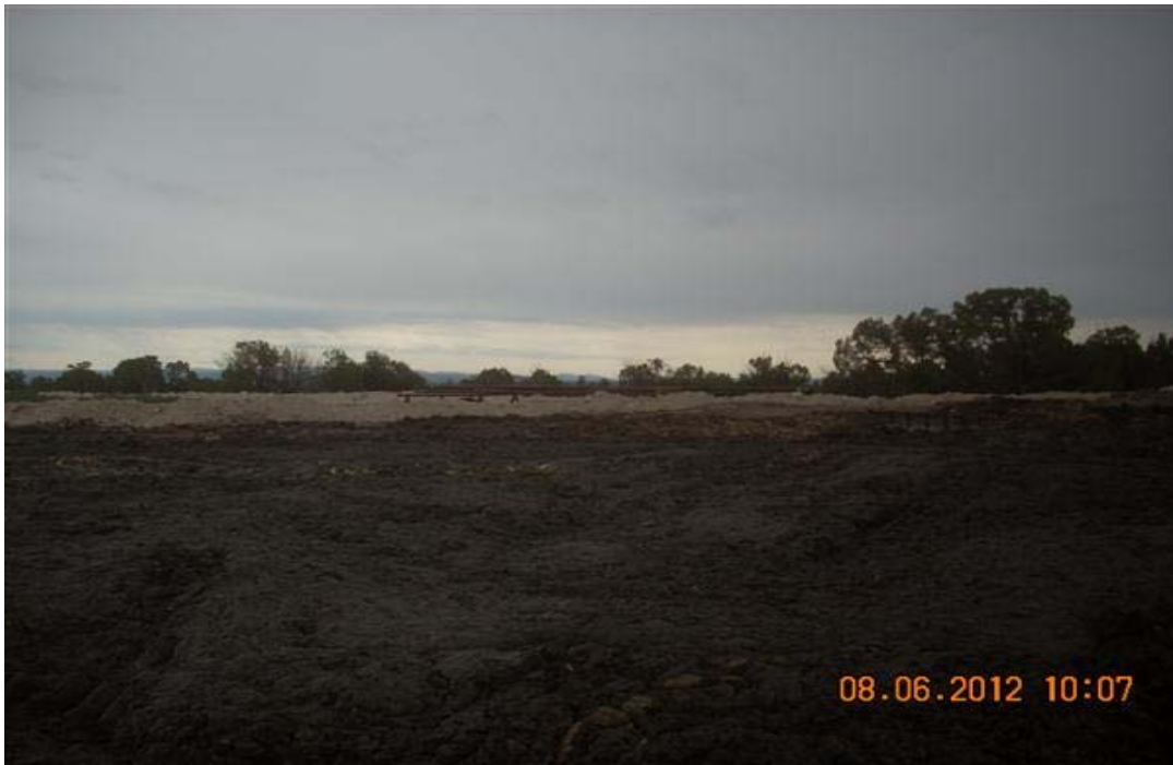
Photo 3 – View of pit contents after removal. Photo taken on 8/6/12.
