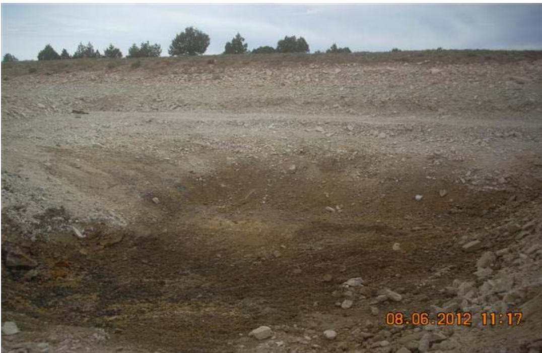
Photo 2 – View of the western end of the pit after removal of the liner. Photo is taken from the southeast corner looking northwest. Photo taken on 8/6/12.
