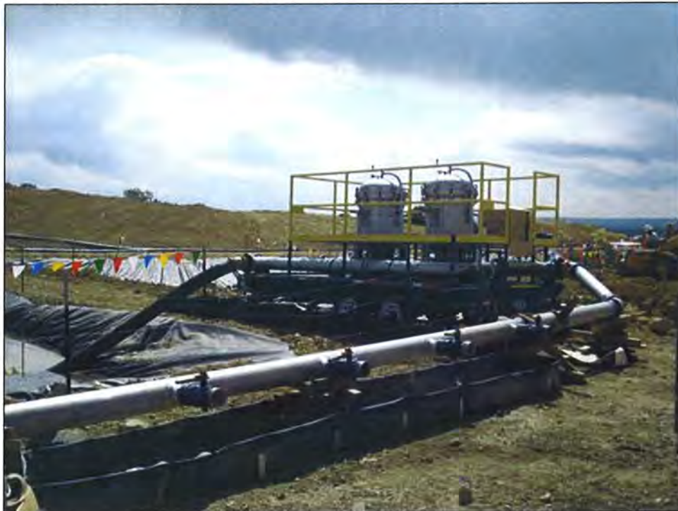
Photo 4. Hose manifold with containment system beneath connections.
