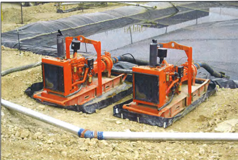
Photo 3. Ecology rails are secondary containment systems that surround the pumps and prevent pump fuel and fluids from reaching the ground.
