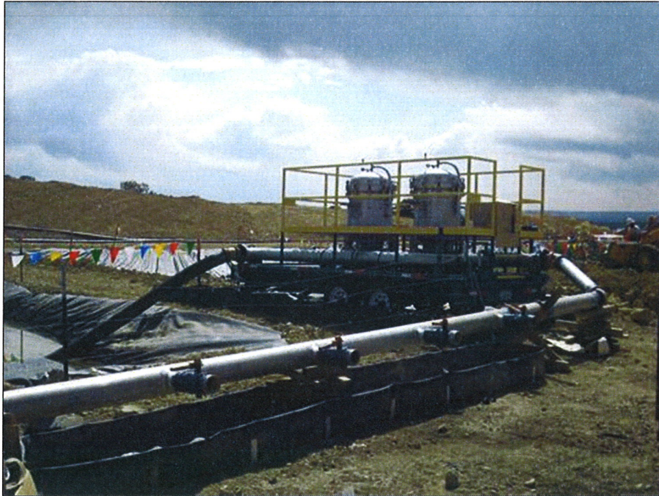
Photo 4. Hose manifold with containment system beneath connections.
