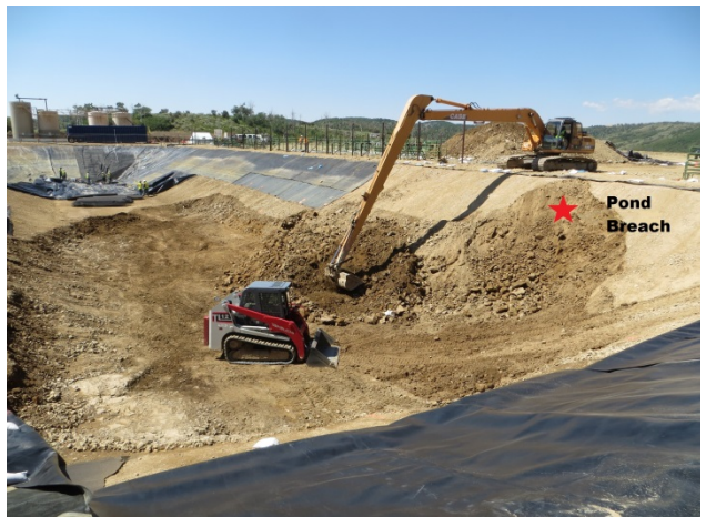
Photo 13 – Looking SW after final excavation of liner breach area
