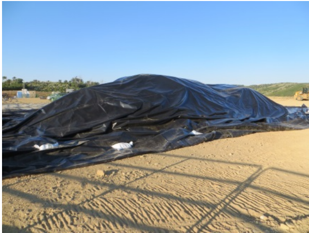
Photo 16 – Cover over plastic-lined waste staging area
