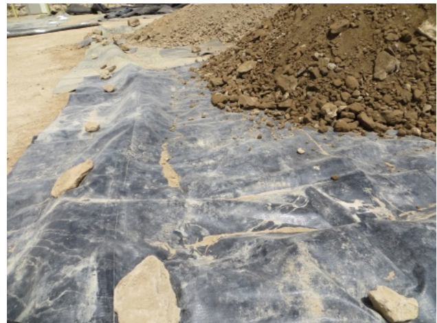
Photo 15 – Berming beneath plastic-lined waste staging area
