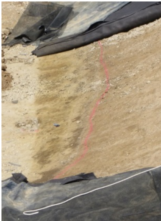
Photo 3 – Closeup of delineation of apparent subgrade contamination
