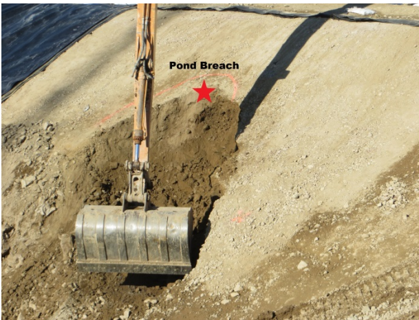
Photo 12 – Looking SW at initial excavation of liner breach area
