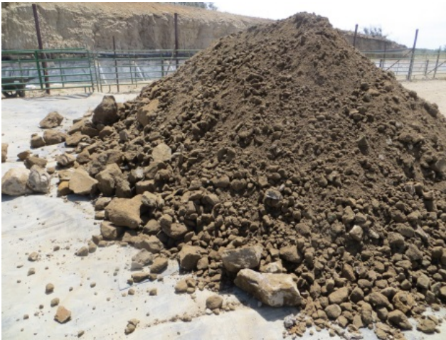
Photo 7 – Contaminated materials staged on plastic liner
