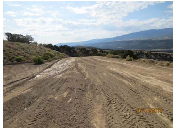
PAD ACCESS LOOKING EASTERLY
