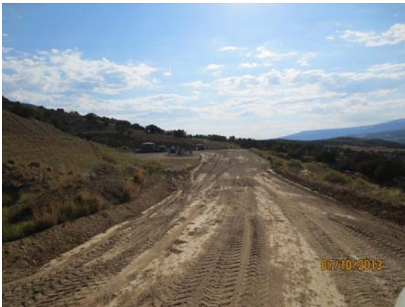
PAD OVERALL LOOKING EASTERLY
