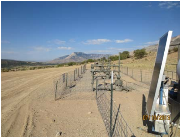
PAD LOCATION LOOKING WEST
