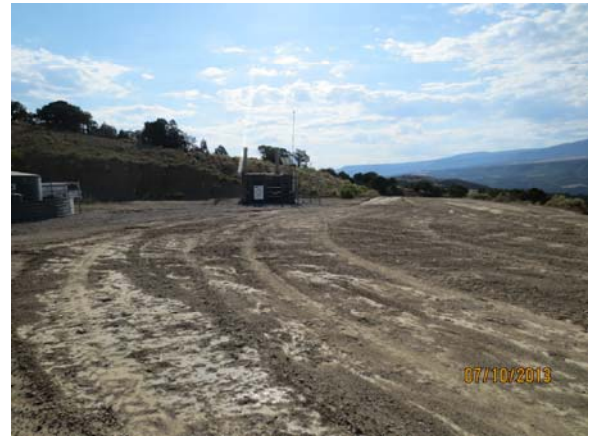
PAD LOCATION LOOKING EAST
