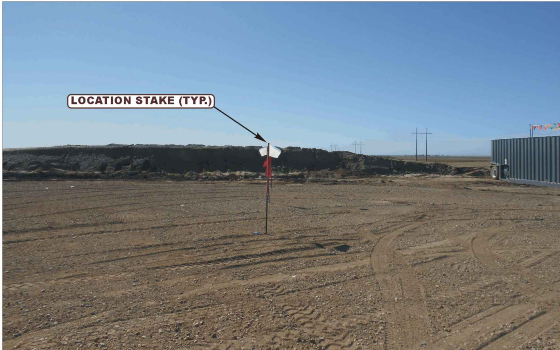
PHOTO: VIEW OF LOCATION STAKES
