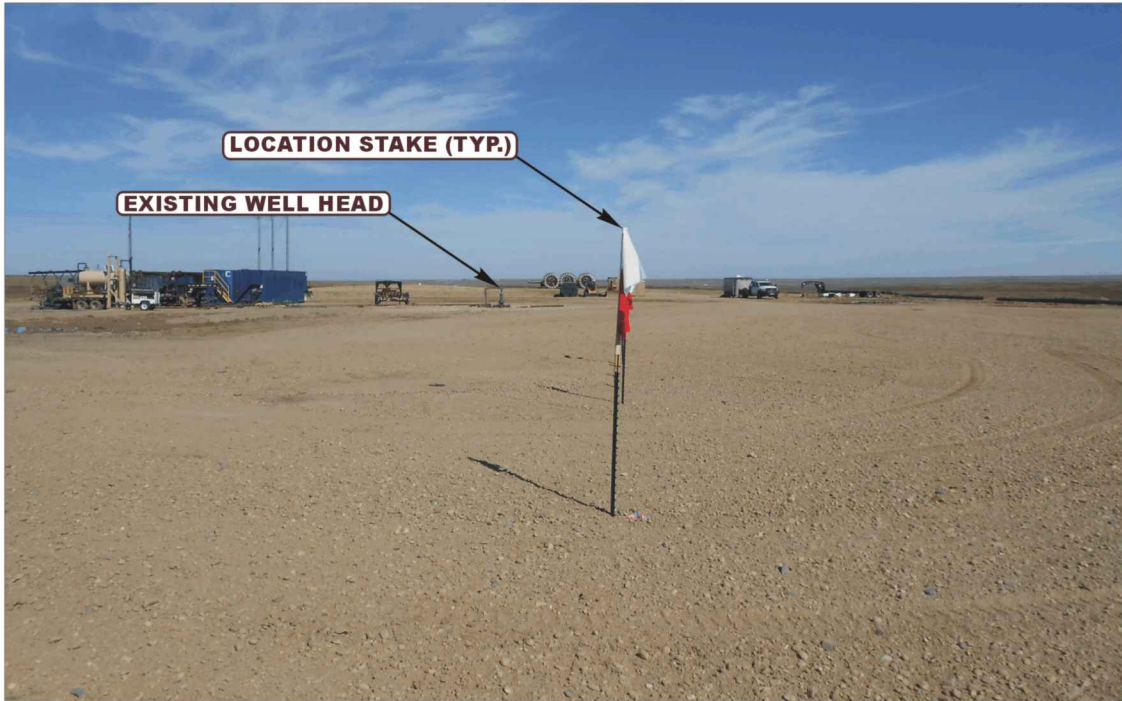
PHOTO: VIEW OF LOCATION STAKES
