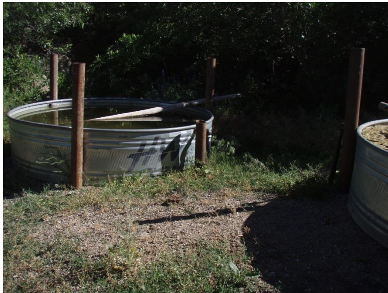
Photo 2. Yellow Jacket Spring; Second Pipe Plumbing to Stock Watering Tanks
