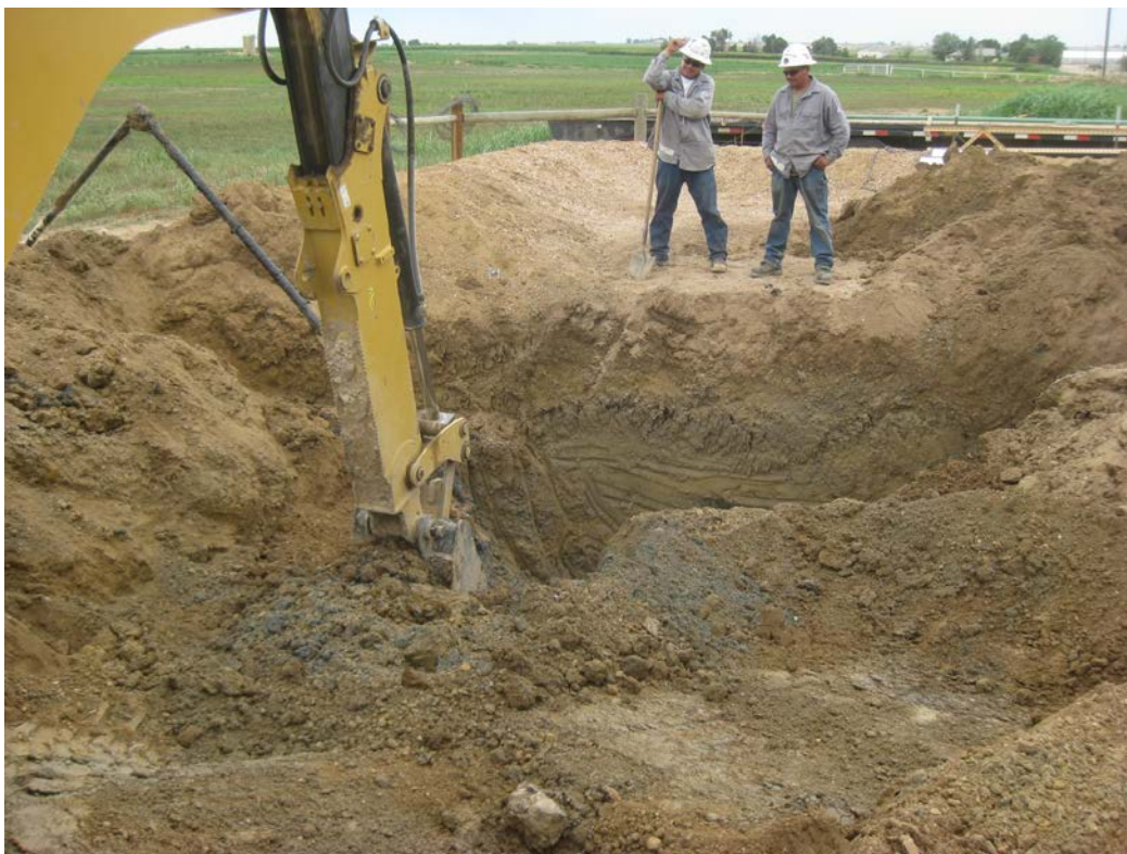
Looking northwest at pit excavation after most of the impacted soil was removed.
