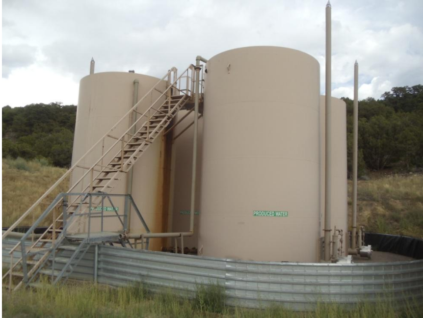
Improper tank labels
