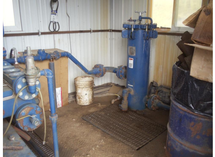
Inside pump house. No secondary containment
