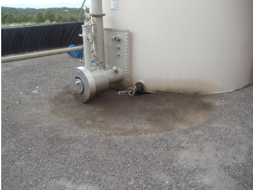
Staining & washout at tank valve
