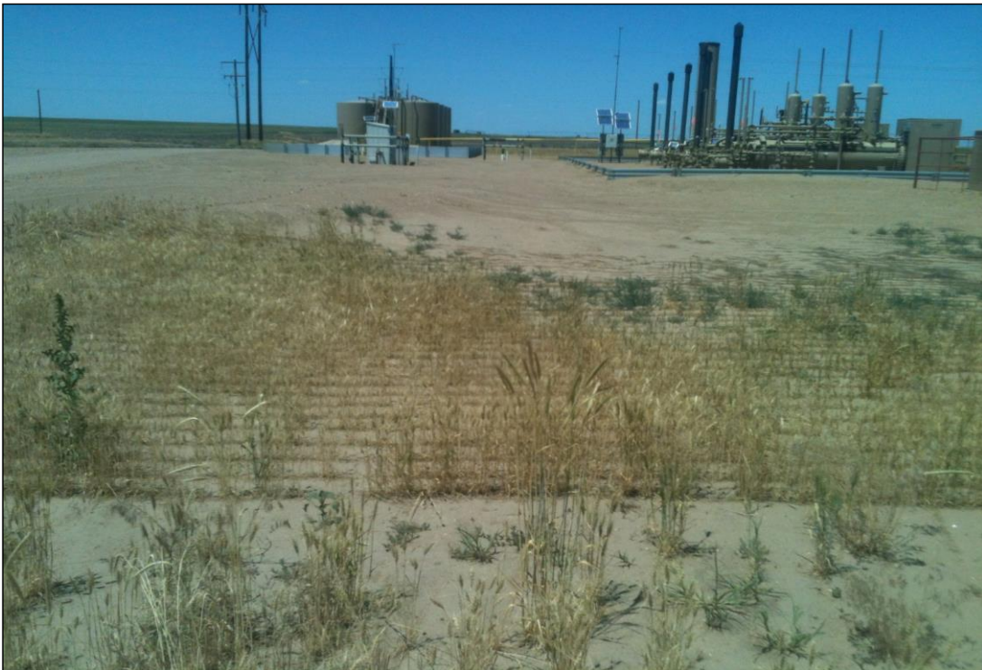
Photograph 5. This is the North facing photograph, as defined in regulation 1003.e.(3). Date Taken: 6/27/2013 GPS Location: 40.15906 -104.68749
