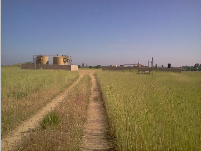
Kugel facilities • North View
