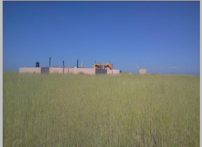
Kugel facilities • West View
