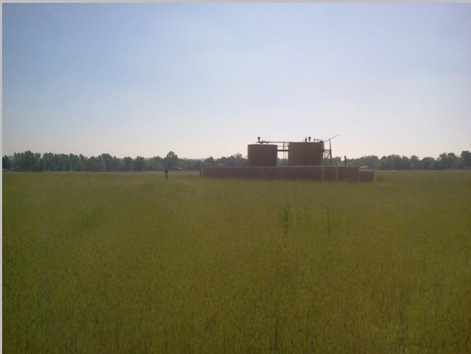
Kugel facilities • East View
