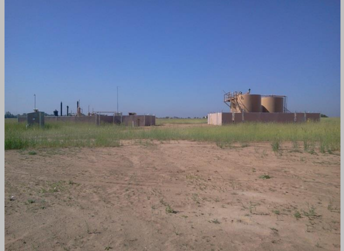
Kugel facilities • South View
