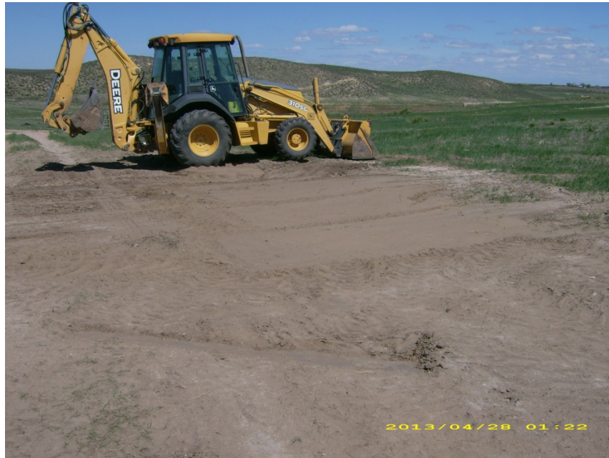
Excavation area after backfilling with clean backfill
