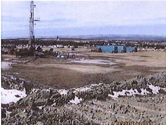
PAD LOCATION LOOKING WEST
