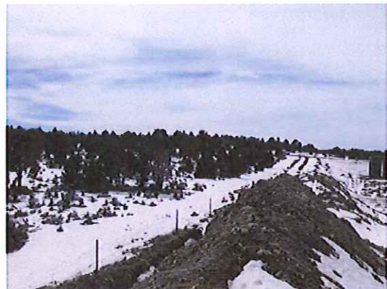
PAD ACCESS LOOKING SOUTHWESTERLY
