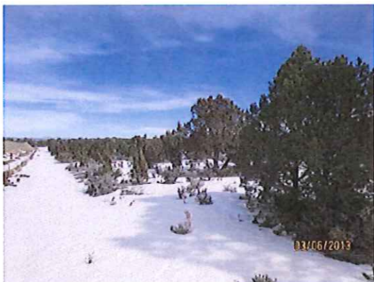
PAD OVERALL LOOKING NORTHWESTERLY
