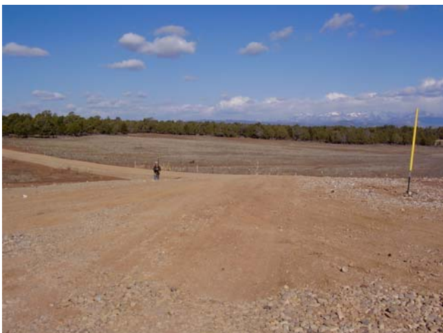
Access at Well Location
