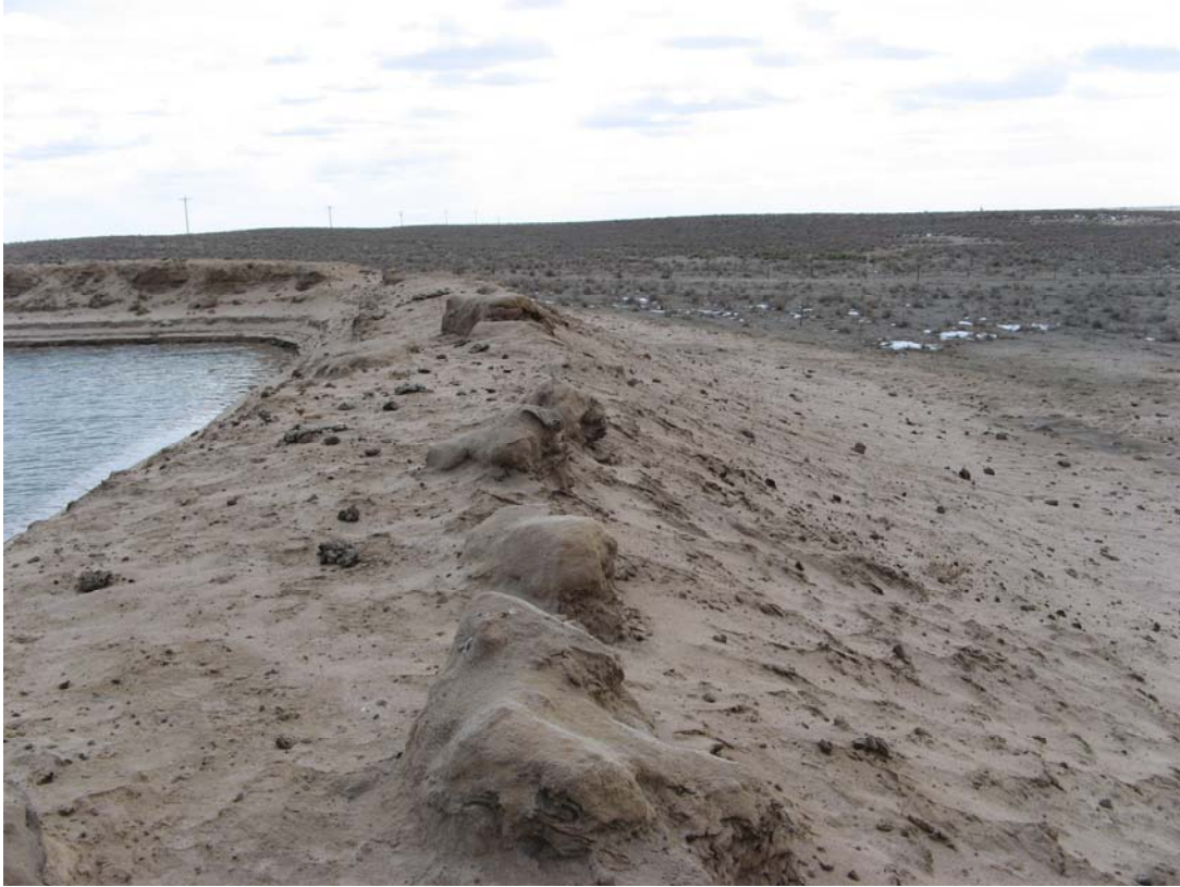
Erosion - west berm water pit looking south
