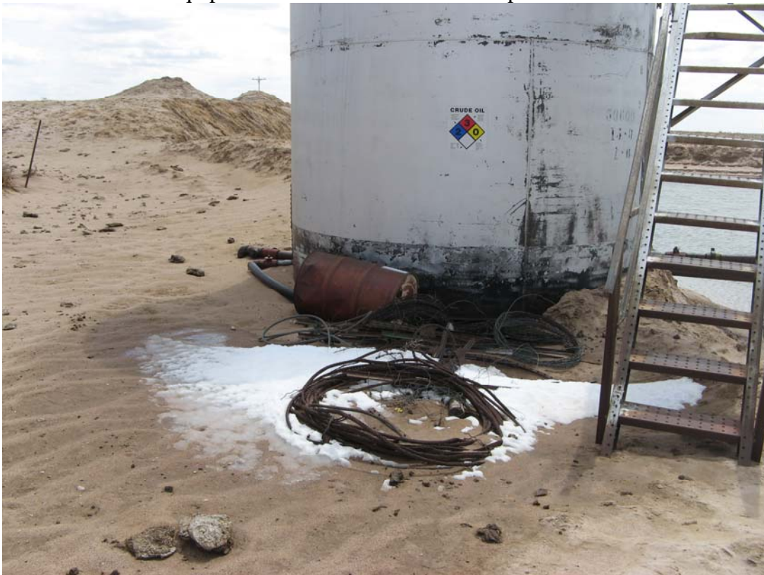
Produced water tank, junk & trash. No berms. Widespread erosion.
