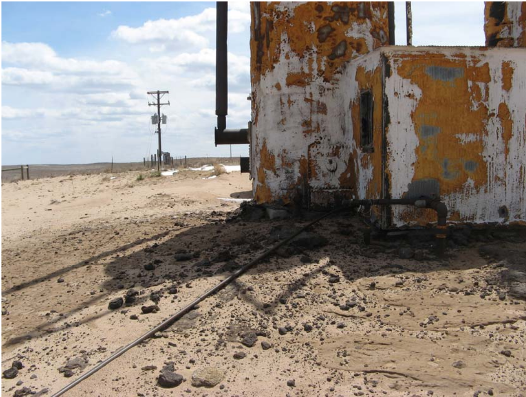
Separator and shed surrounded by oily waste.
