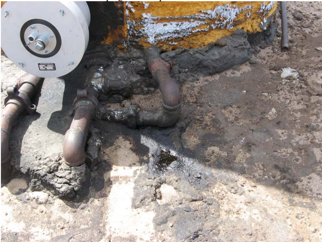
Dripping equipment at battery
